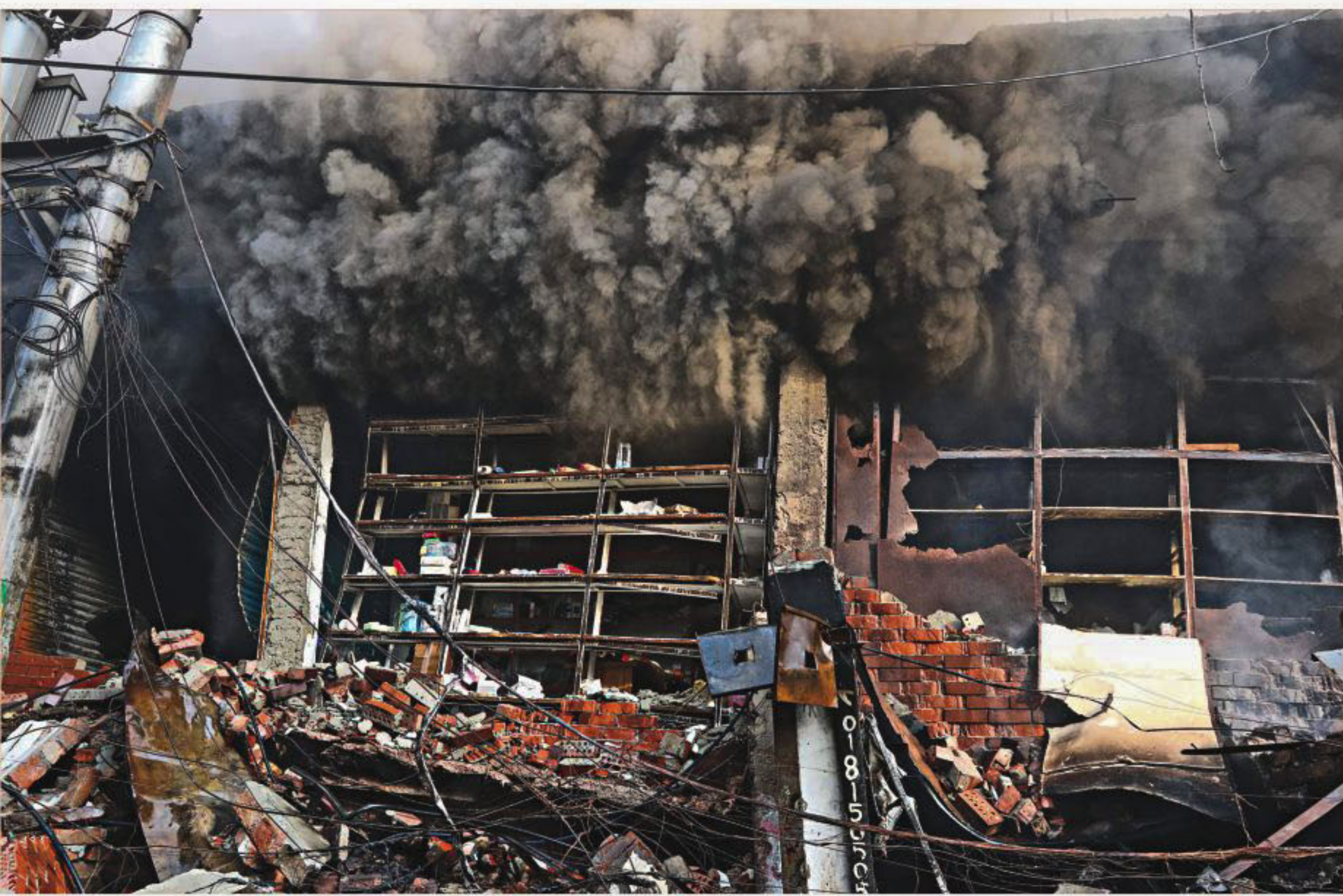
Smoke billows from the Gulshan-1 DCC Market in the capital yesterday. The market partially collapsed in the blaze. More photos on page 3.
