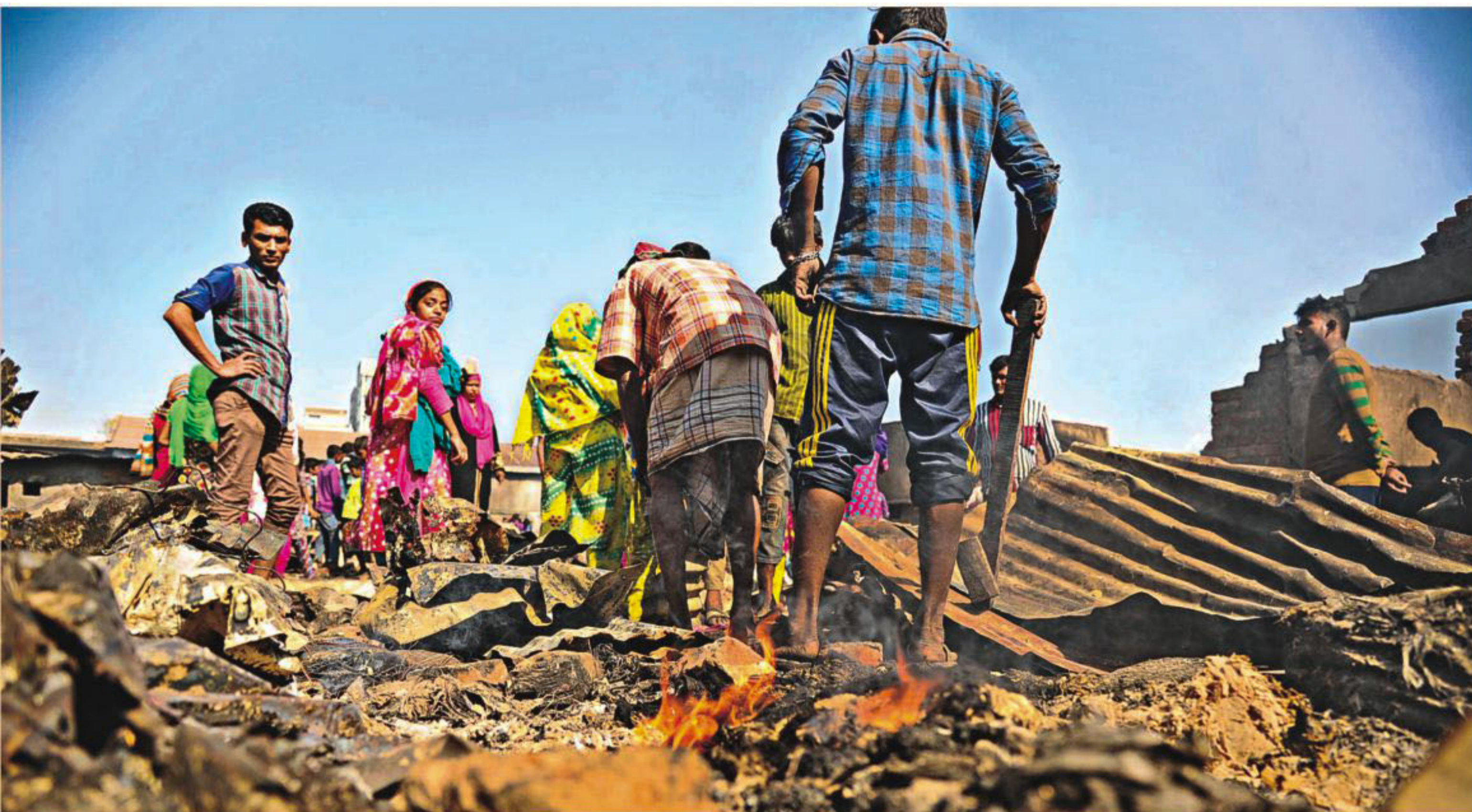
Debris being cleared after a fire, as per firefighters, originated from an electric short circuit in a house at the Maillar Bil slum in Chittagong city's Sadarghat area early yesterday, gutting 20 houses and six shops.
