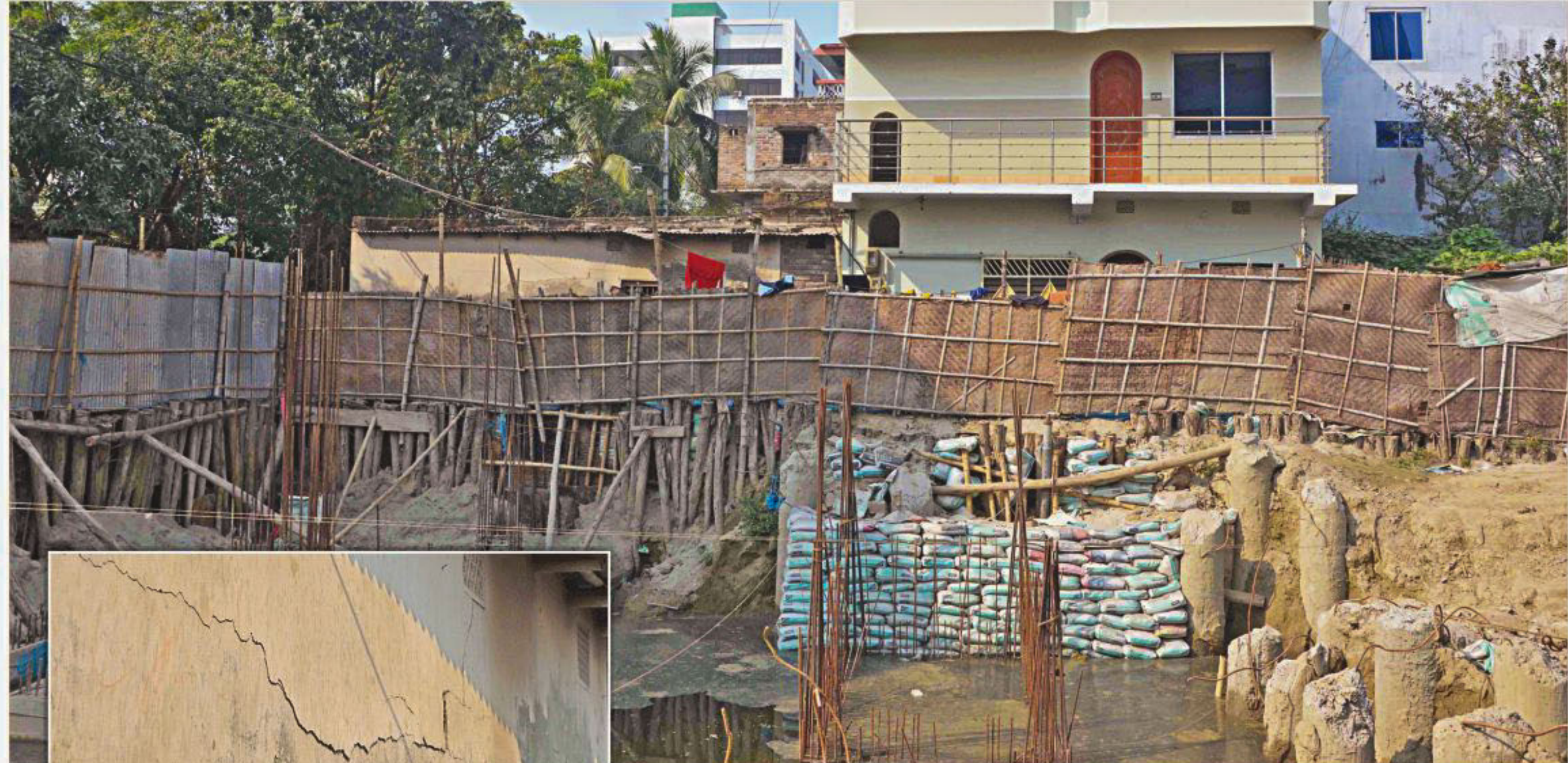
A foundation pit dug for construction of a 16-story building in Rajshahi city without approval. The illegal construction caused the adjoining three-story building to tilt and a one-story building to develop cracks., inset. PHOTO: AnWAR AII
