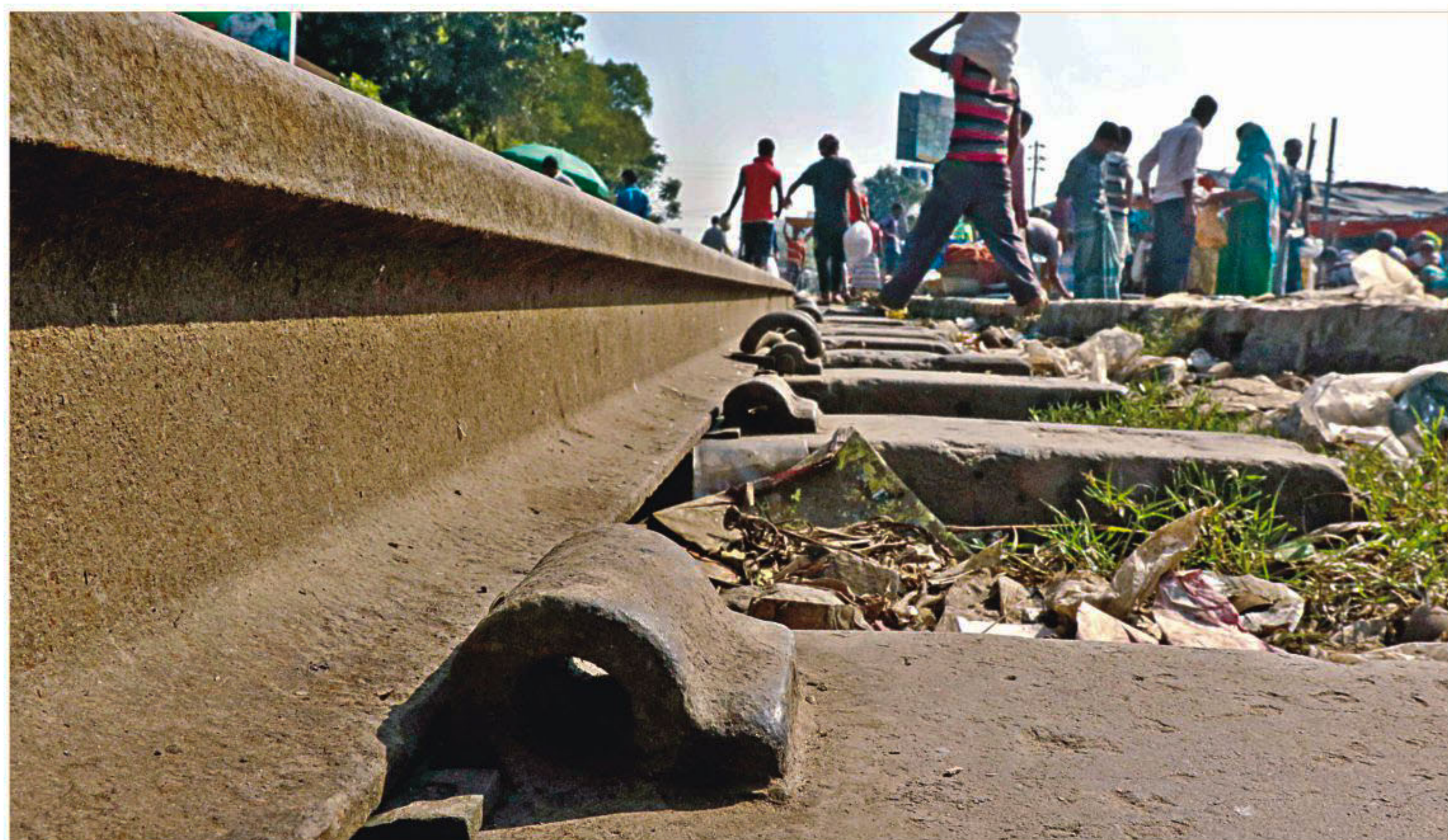
Tracks missing their rail anchors near the fish wholesale market in the capital's Kawran Bazar. There are over 100 missing in the stretch from here till the Moghbazar crossing. Locals say drug abusers break these off to sell at metal recycling shops for Tk 40 a kilogramme. The photo was taken last month.
