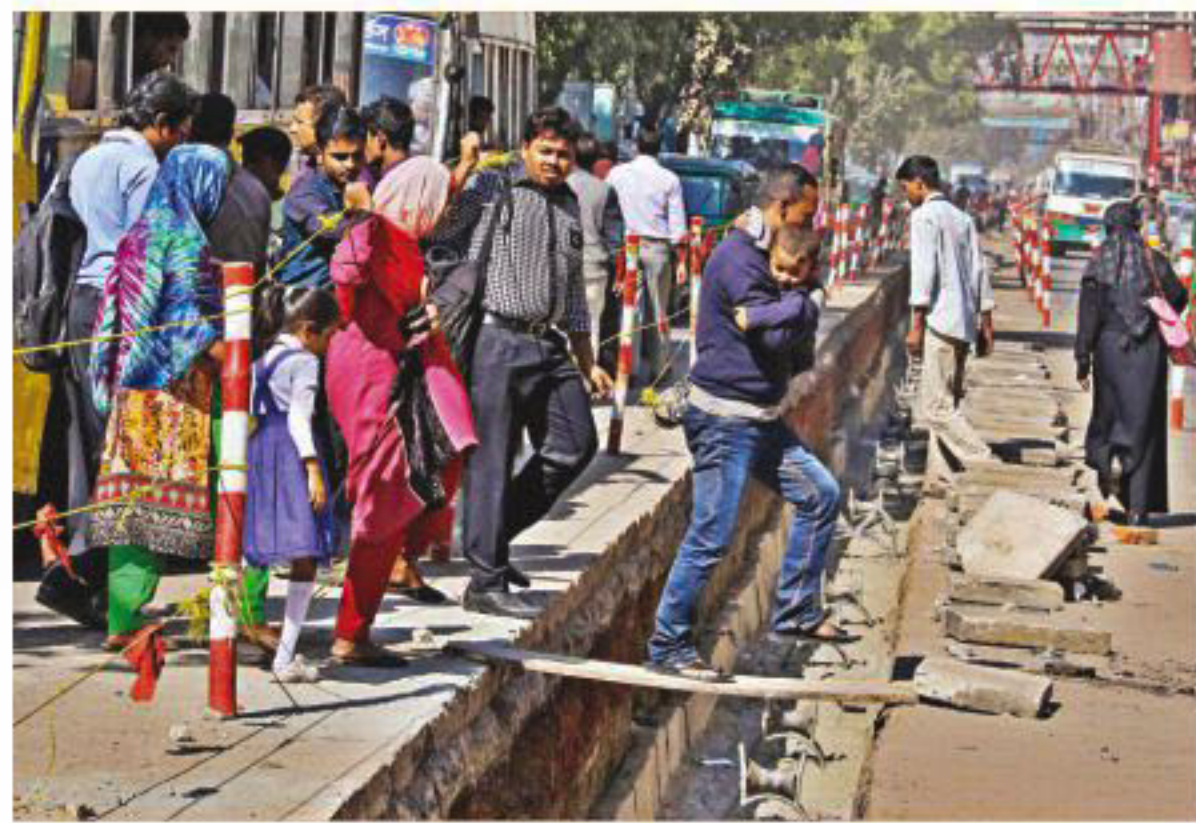
Utility lines being laid on Rokeya Sarani, on the stretch from Agargaon to the Mirpur 10 roundabout, in the capital as part of the construction of metro rail yesterday. Since the rearrangement is to go on till February before the excavation shifts to Pallabi, vehicles bear the long, slow queues and the absence of hard barriers while people the dirt and risks to get on with their daily lives.
