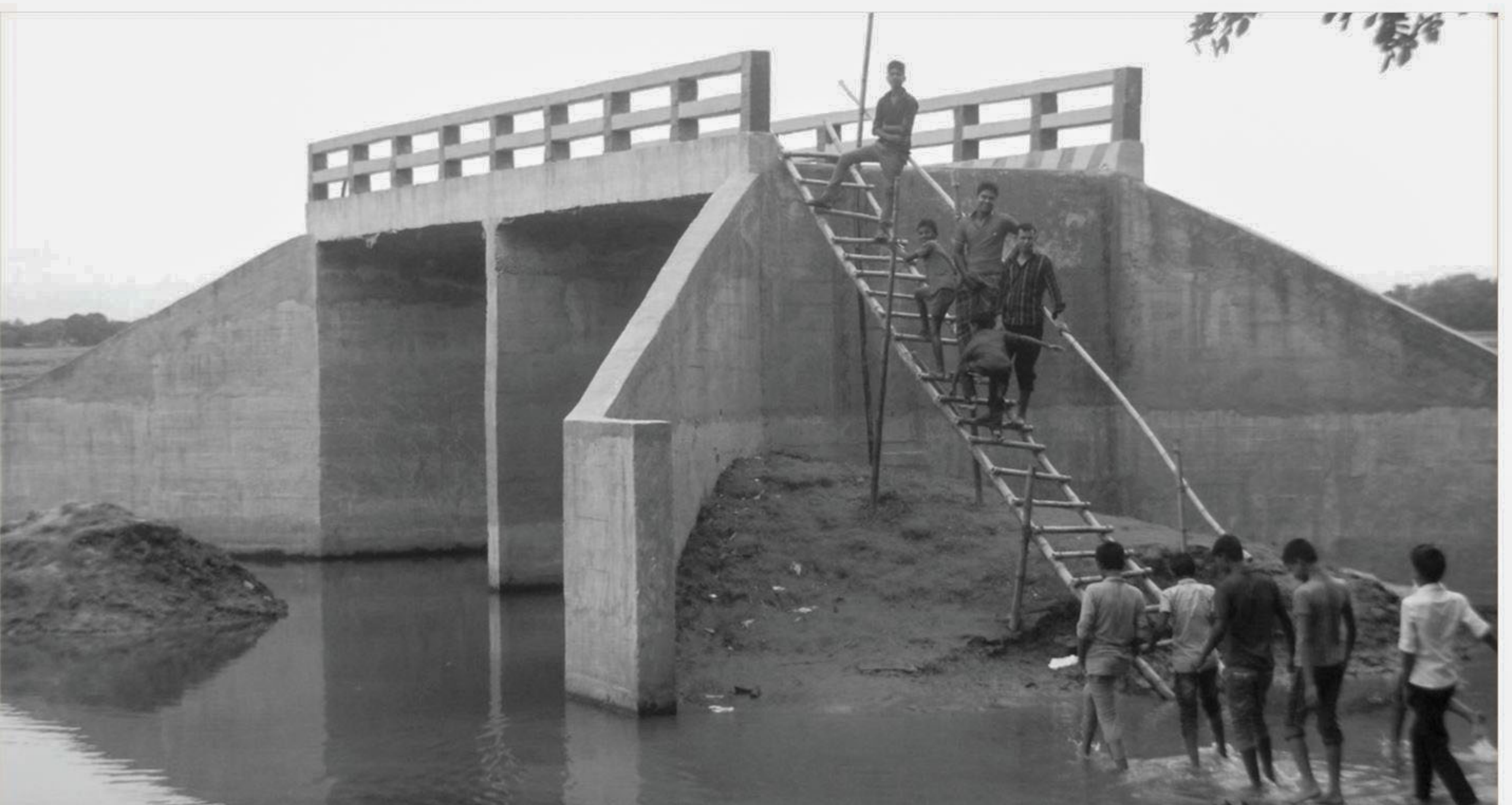
BRIDGE INDEED: People use a bamboo ladder to get on and down from the bridge on the Kharia river at Rambhadrapur in Phulpur upazila of Mymensingh as the bridge, too small for the width of the watercourse, also lacks approach road.
