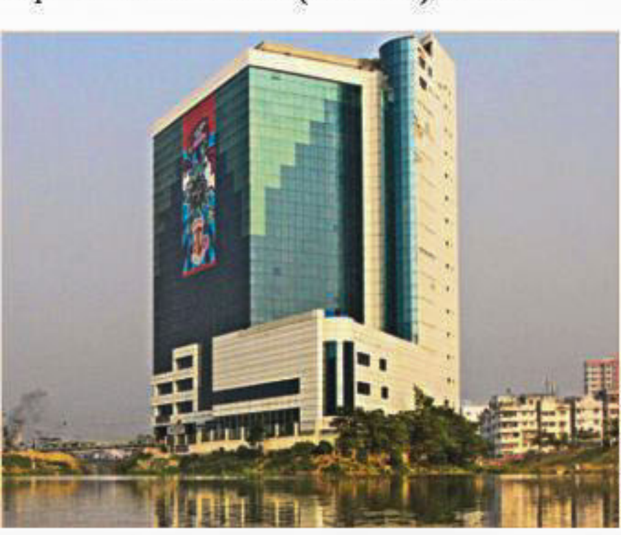
"BGMEA Complex" on Begunbari canal.
