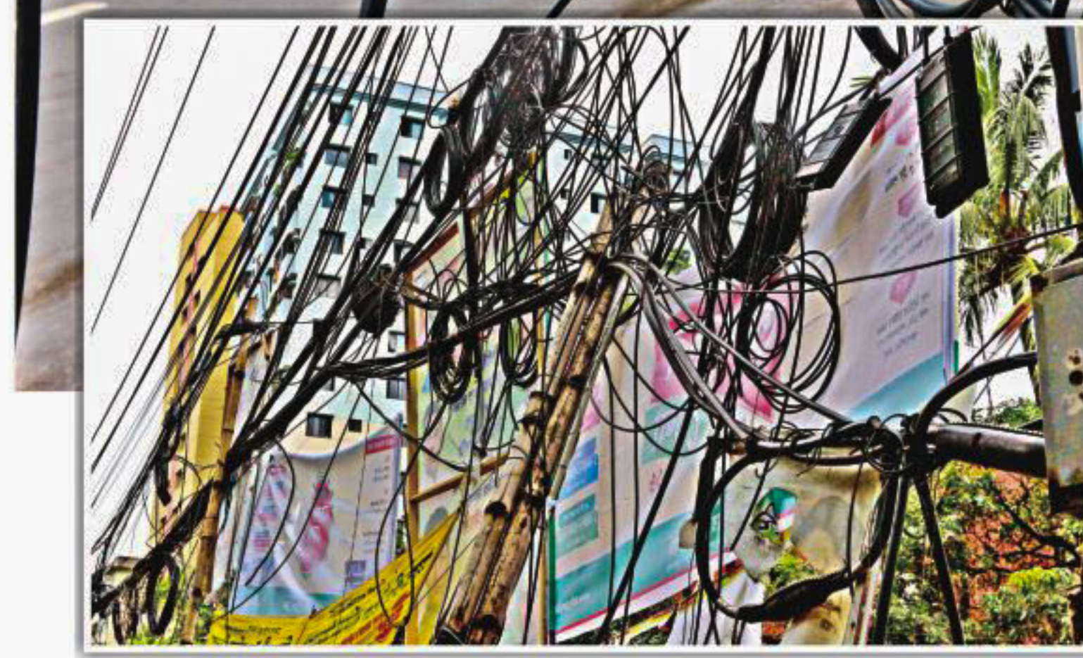
Strung on free standing bamboo poles at eye level, these cables carry power, internet and cable TV service and tell a tangled tale of the failure of the authorities to enforce regulation and ensure safety to the residents of the mega city. The photo was taken yesterday at Segunbagicha.
