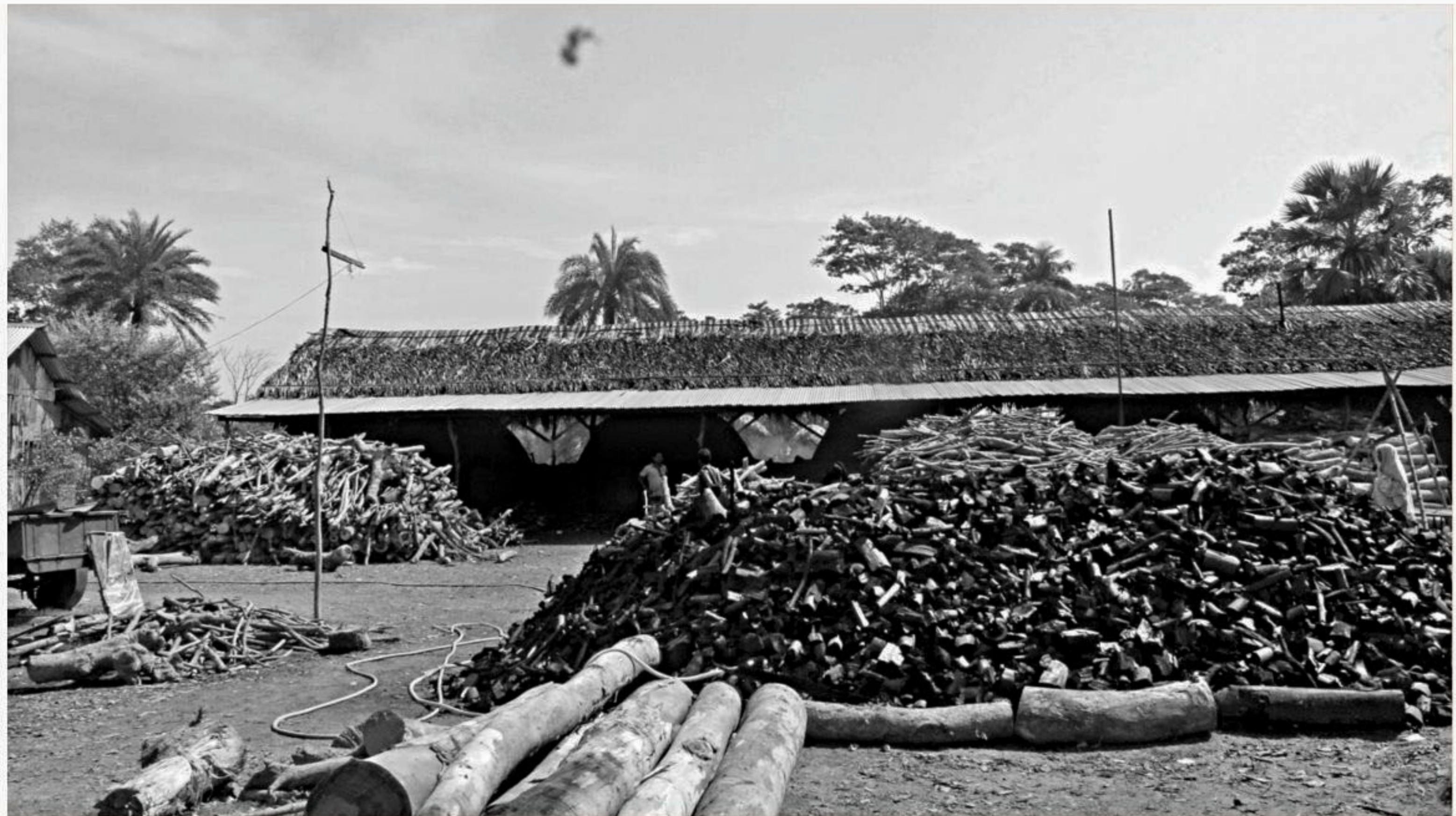
An illegal charcoal plant built by a Jubo League leader on waqf land in Kalaiya village of Baufal upazila under Patuakhali.
