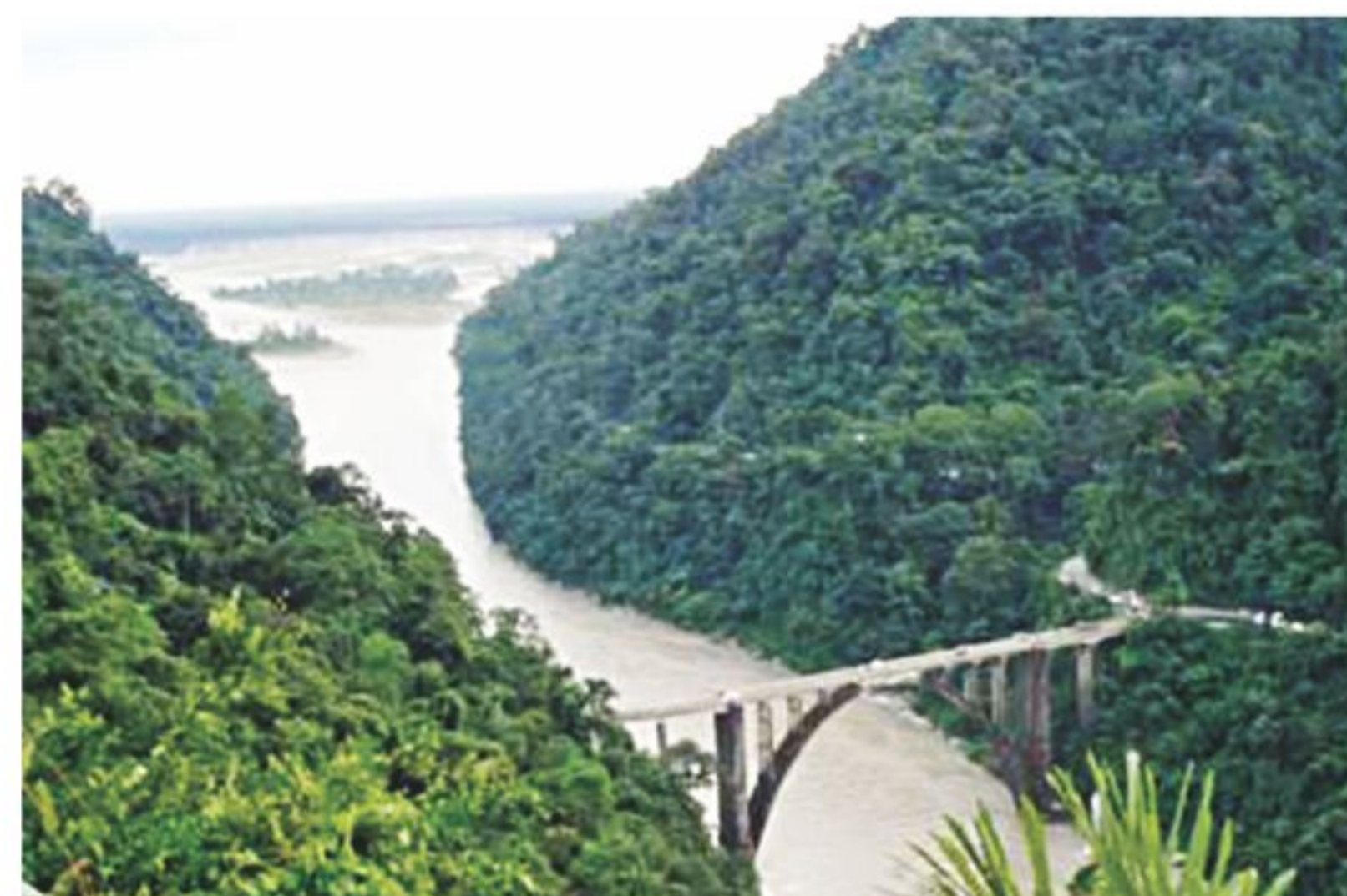
Coronation bridge built in 1941, 20 kms away from Siliguri
