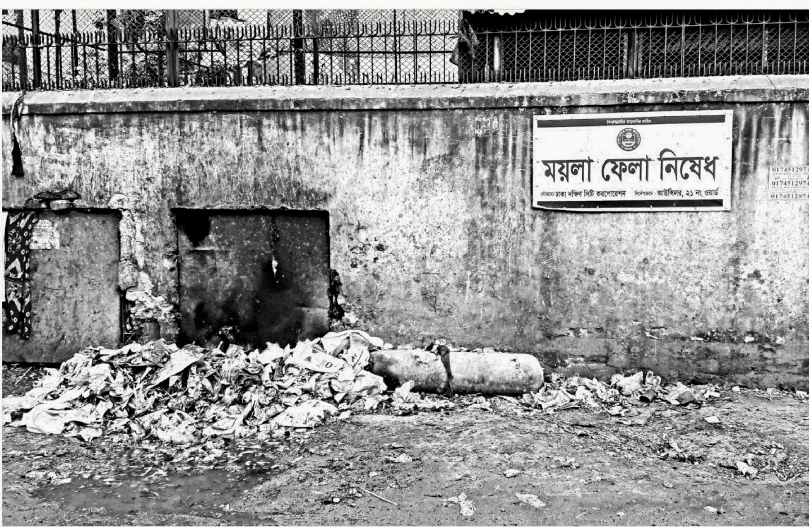
Despite the presence of a glaring signboard hung up by Dhaka South City Corporation asking people not to dump waste there, they keep dumping trashes by the road, yards away from the west gate of Bangabandhu Sheikh Mujib Medical University in the capital. The photo was taken on Wednesday.
