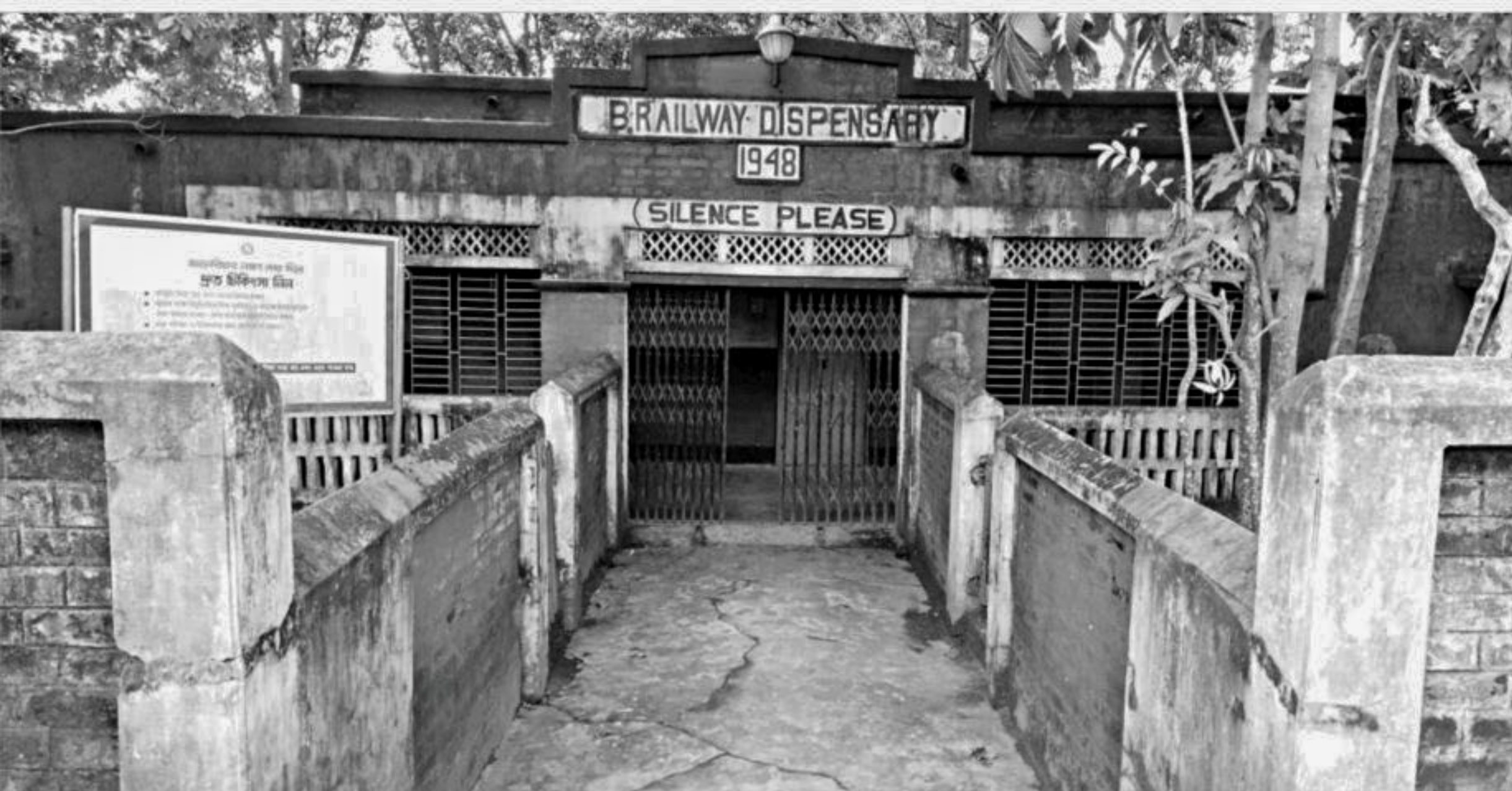
Kulaura railway dispensary in Moulvibazar. The photo was taken recently.
