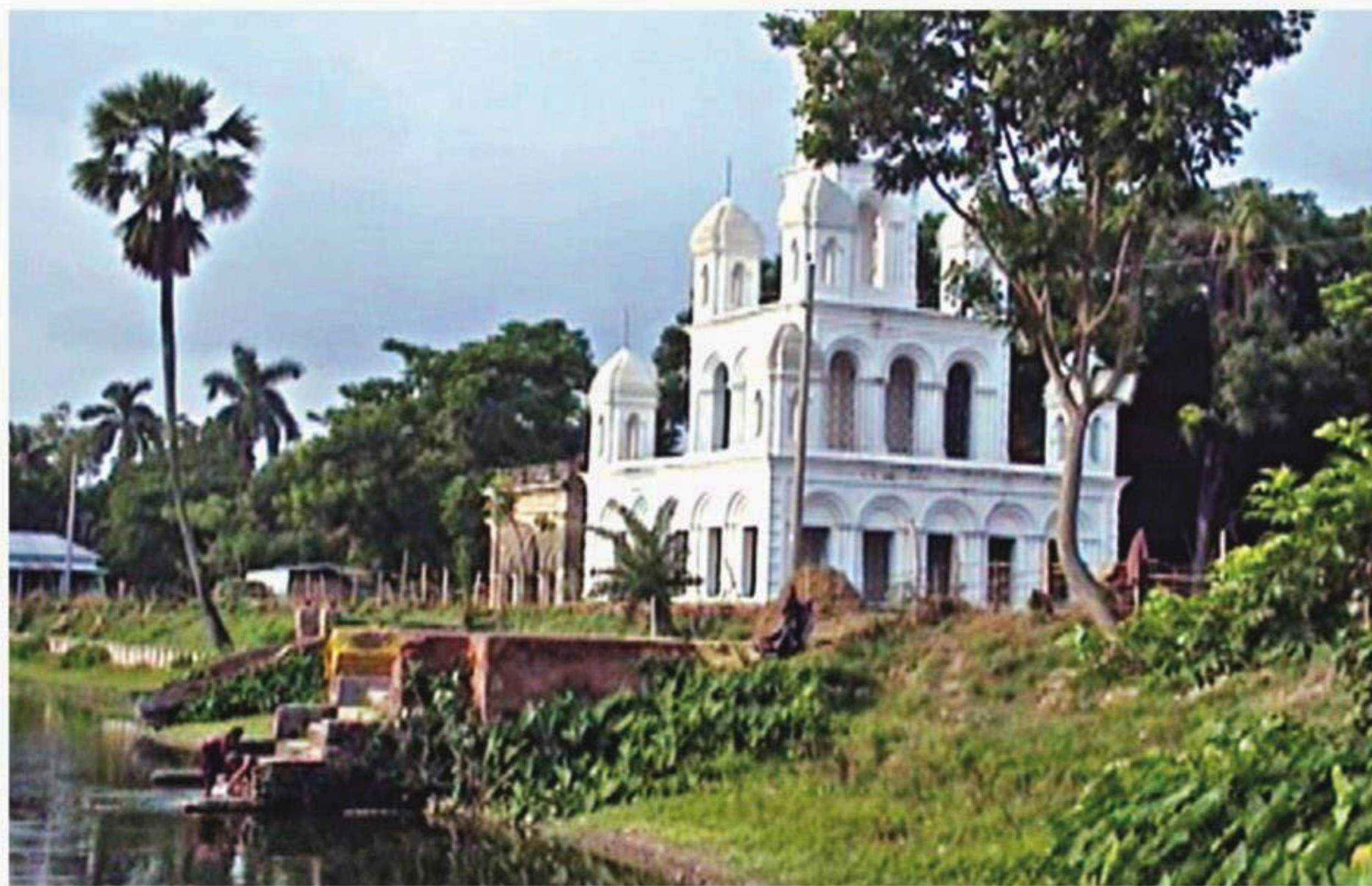
The renovated Navaratna Math on the premises of the Teota Palace in Manikganj's Shivalaya upazila. Right, part of the dilapidated palace. The photos were taken recently.
