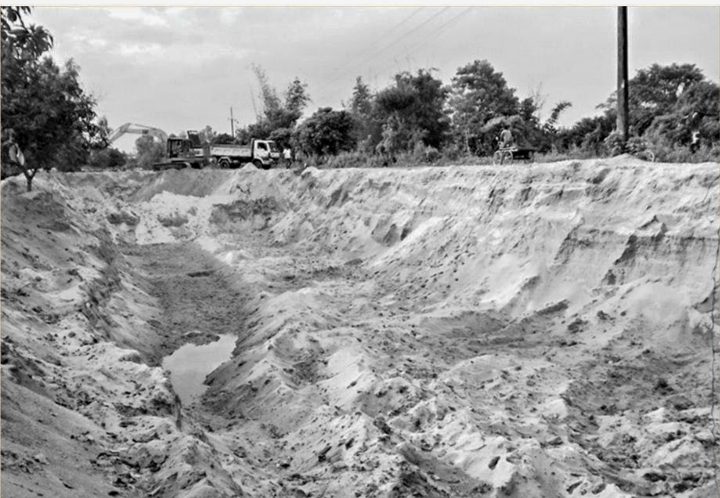
A road in Phulbari upazila of Dinajpur is on the verge of collapse as this large pit has been created next to it due to illegal sand lifting by a local influential person.
