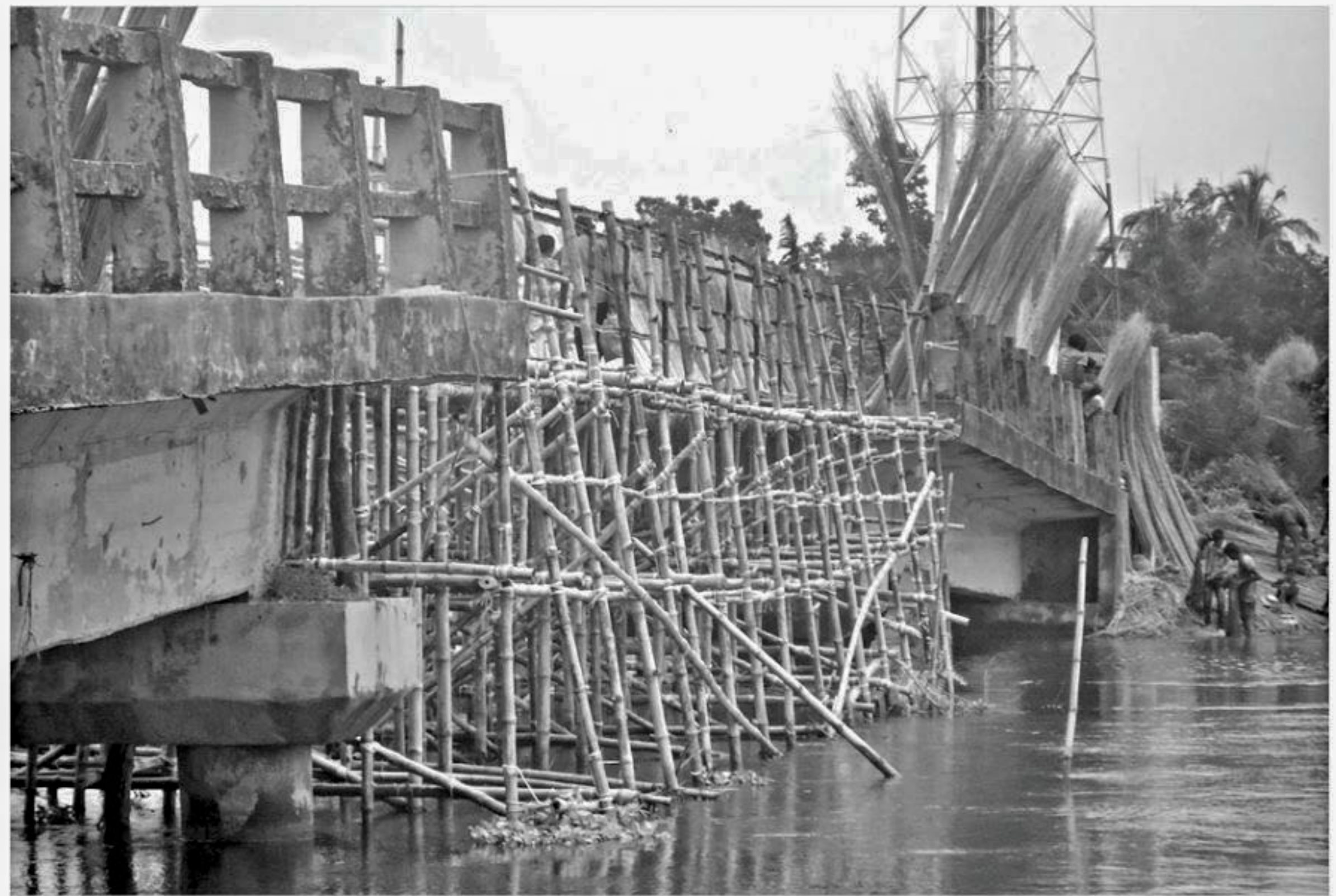
Local people erect a bamboo bridge on their own as a replacement for the middle section of the concrete bridge on the Sanchai river in Jhenidah that collapsed suddenly on June 6 this year.
