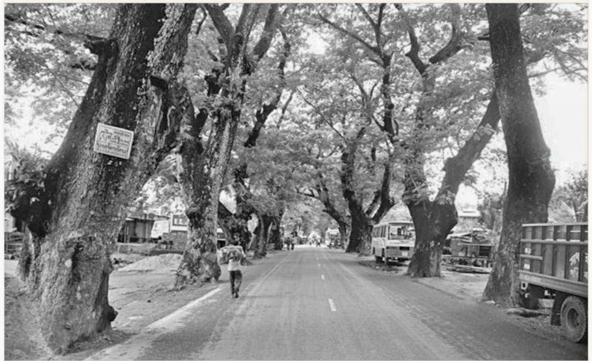
Work for turning the commercially important Benapole-Jessore highway into a four-lane road is going to start soon, much to the happiness of traders and other stakeholders.
