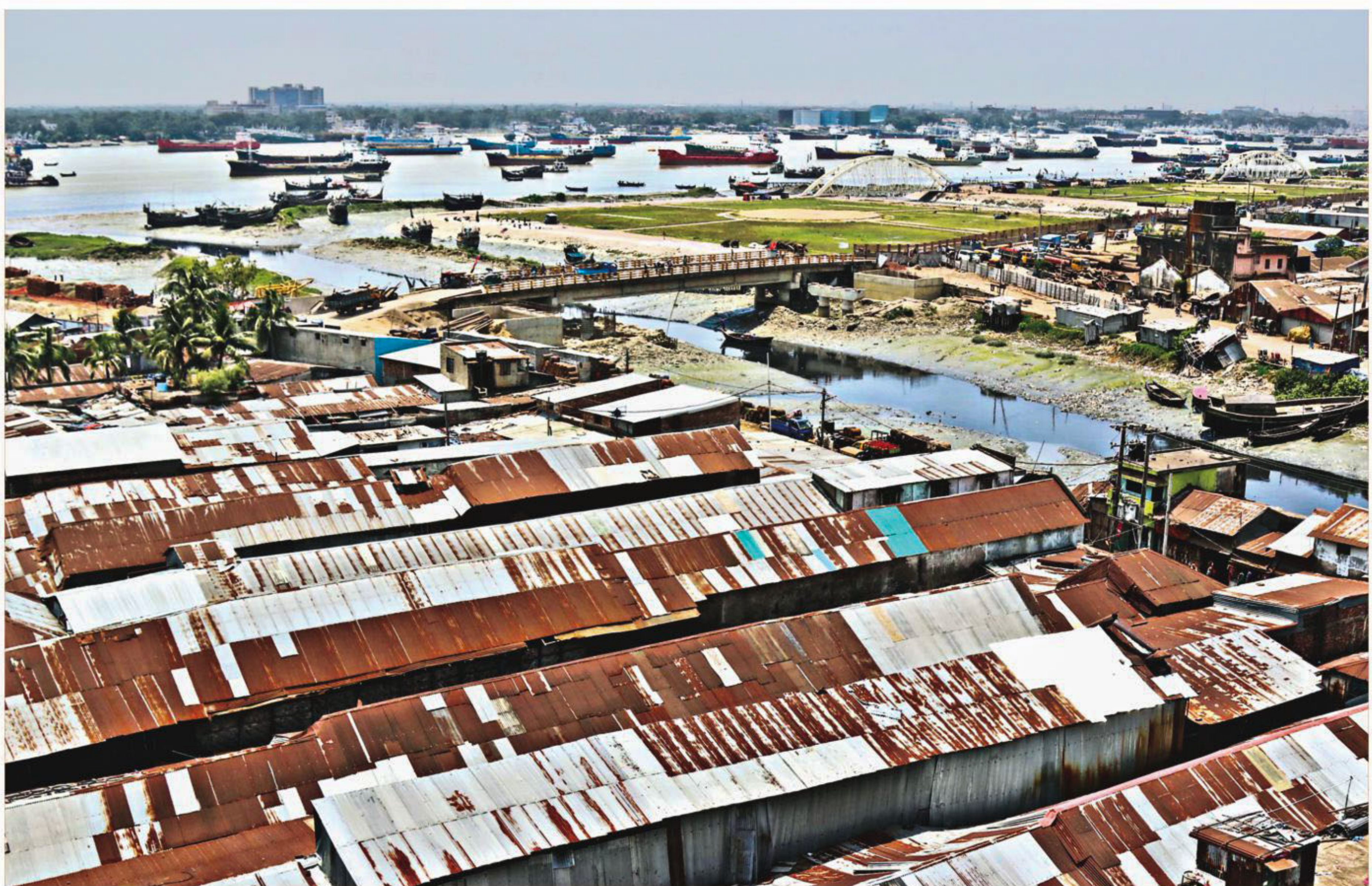
Illegal structures line a 22km stretch of the bank of the Karnaphuli River in Chittagong city. These grew up over the last 90 years since 1927. Six years after a rights group filed a writ petition, in 2010, the High Court last month gave an order, asking the district administration to evict the encroachers.
