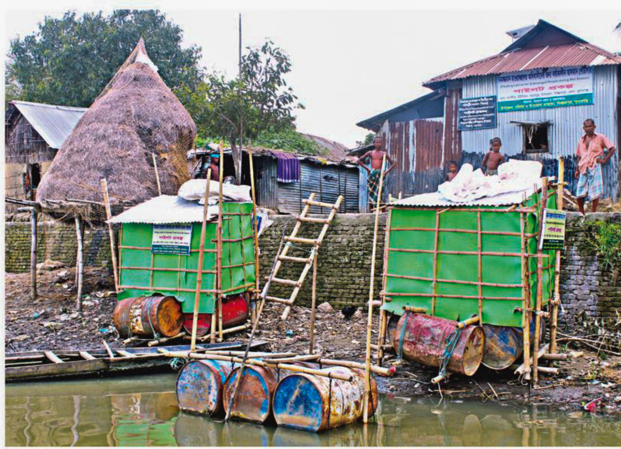
Special floating toilets in Sunamganj's Bishwambarpur upazila. The toilets, invented by the upazila's former assistant commissioner for land Muhammad Talut, bottom right, are meant for ensuring hygienic sanitation for haor people.
