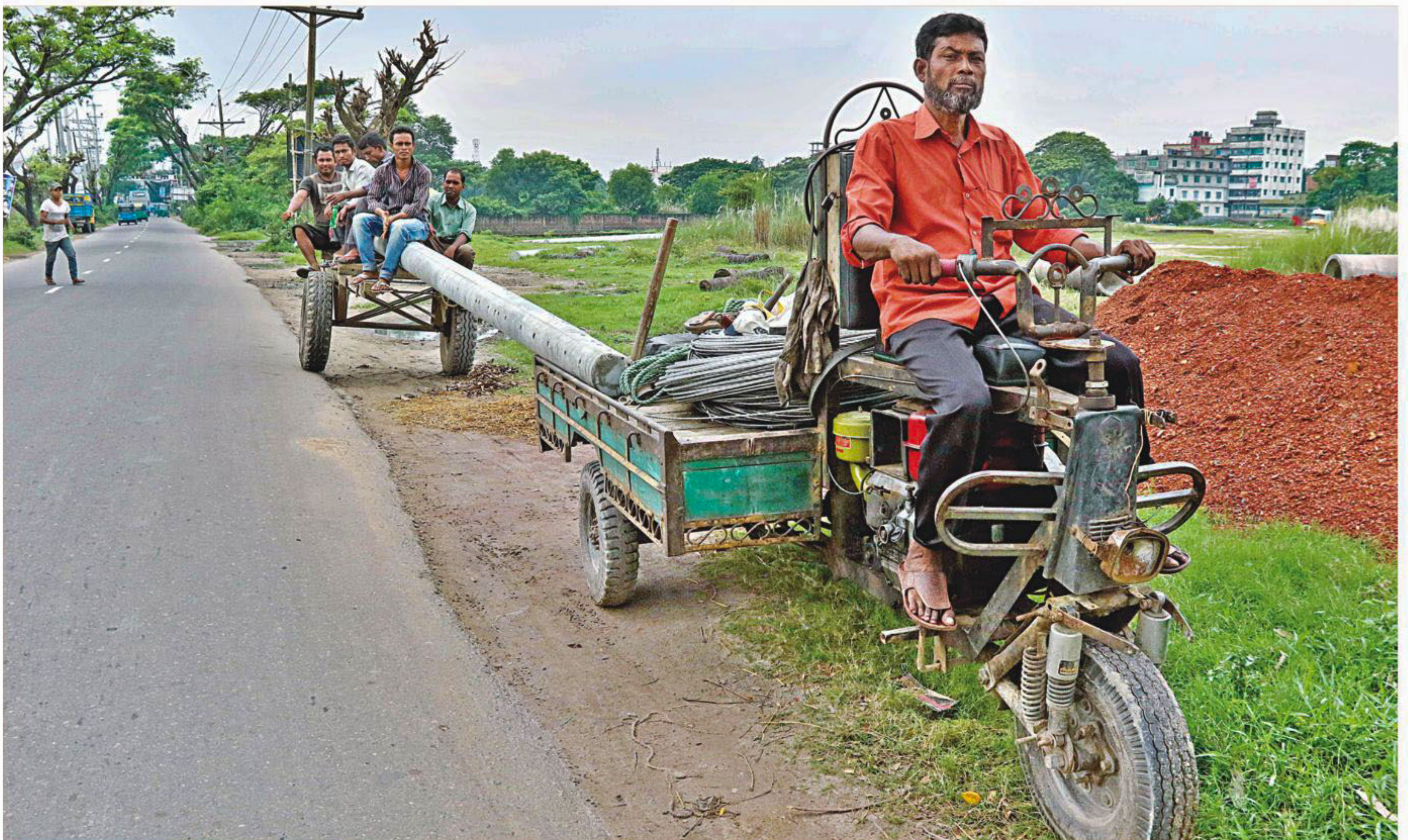
Ignoring risks of accidents, a contractor transports an around 50-foot concrete electricity pole, precariously placed between a Nosimon, an improvised three-wheeler, and a pushcart on the Keraniganj-Dohar road. The contractor resorted to the hazardous process because Bangladesh Rural Electrification Board, which hired him, did not have a vehicle suited for the job. The photo was taken at Godarbagh Konakhola, Keraniganj on Tuesday around noon.
