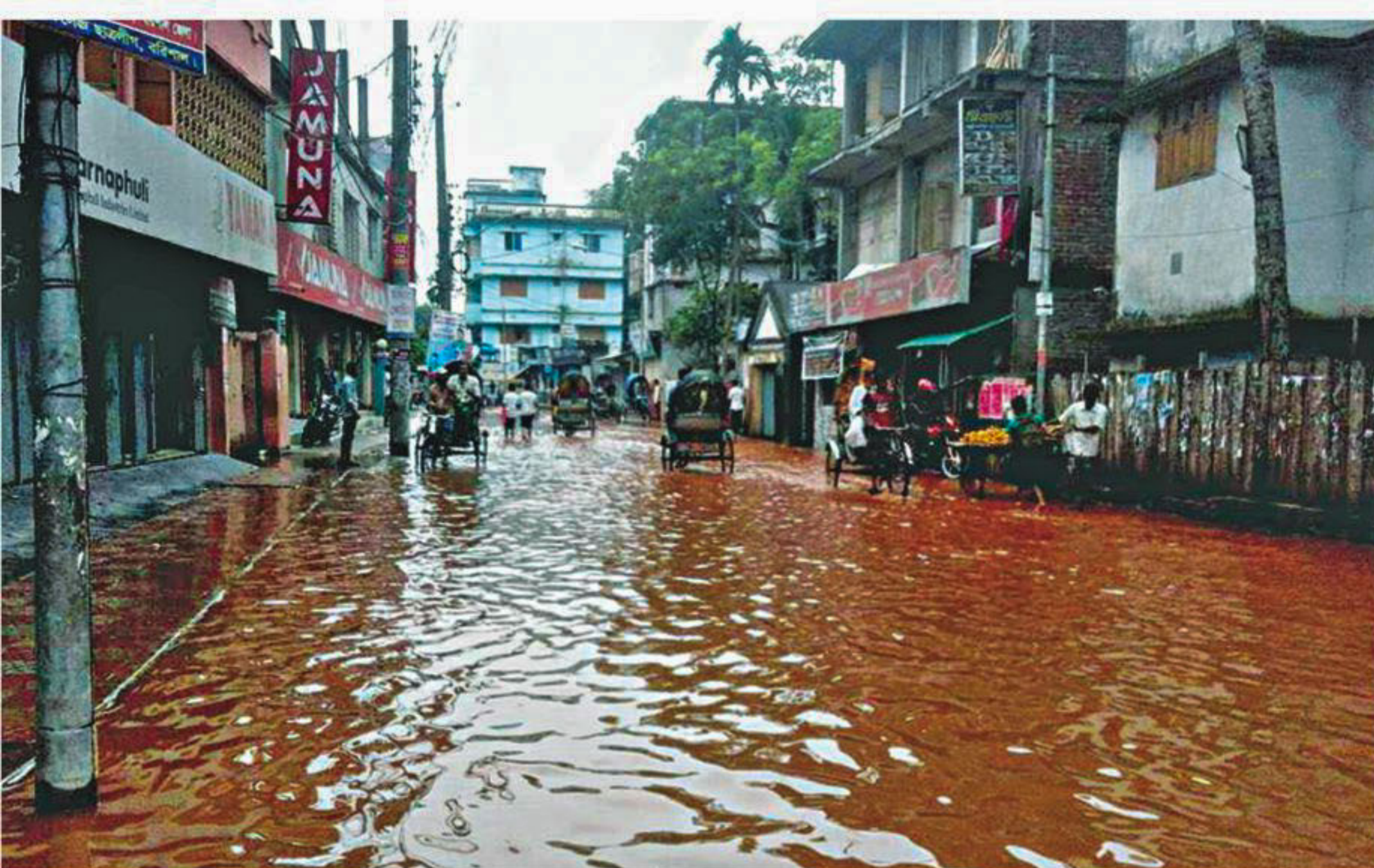
The brick-built Jibanananda Das road in Barisal city after heavy rain yesterday, for which most of the low-lying areas of the city went under water. Clogged and inadequate drainage system and filling up of most of the canals are mainly responsible for such waterlogging, compounding miseries of the residents.
