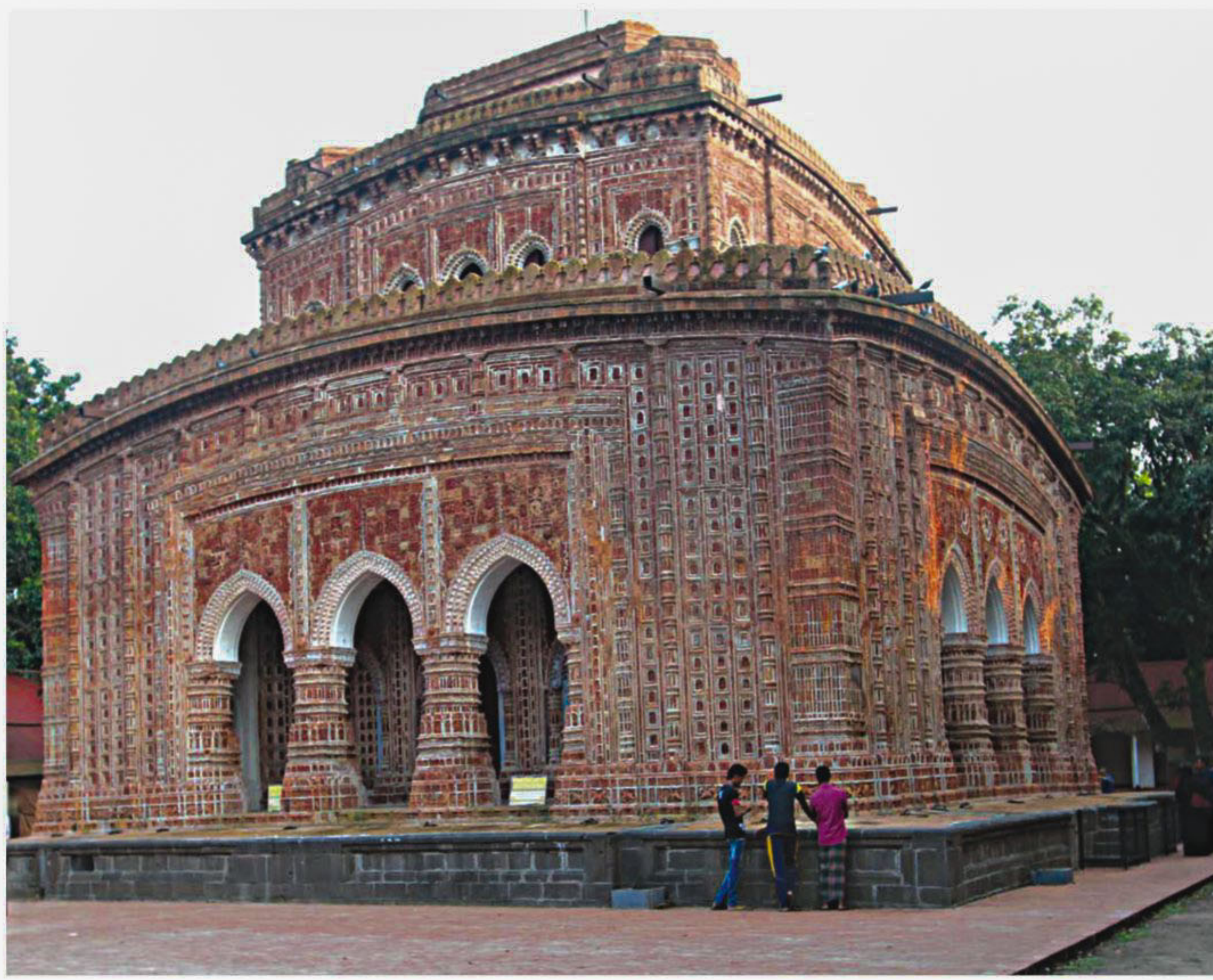
The stunning Kantaji temple in Dinajpur after renovation. Restored terracotta carvings on top right, and worn-out terracotta works, middle and bottom, before the restoration and site development began in August last year.
