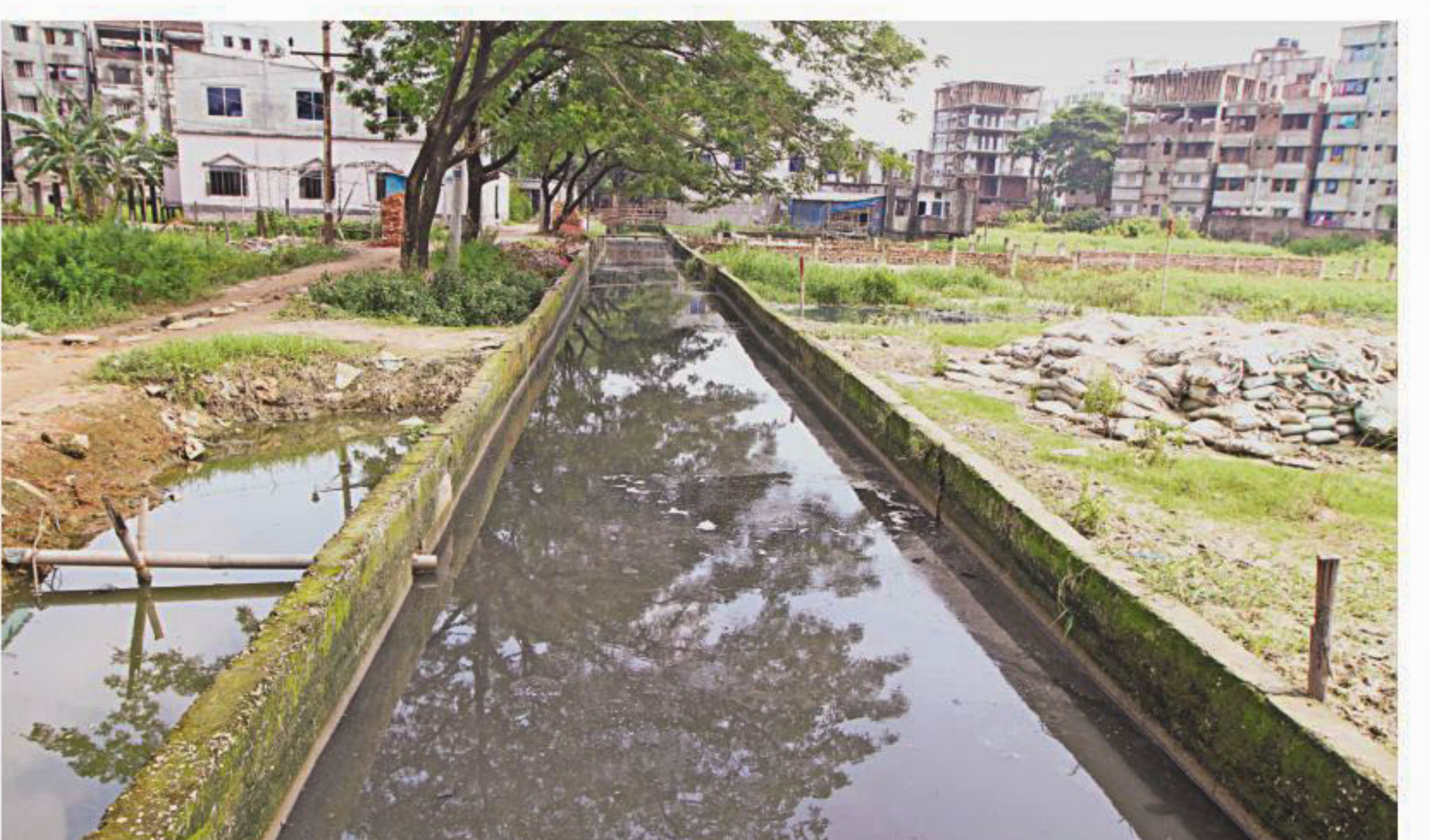
Left, the lining work at the sides of the Ibrahimpur canal has not only reduced its width but also made it a garbage destination, while the U-channel work on the Gerani canal has narrowed down its width reducing the water carrying capacity.
