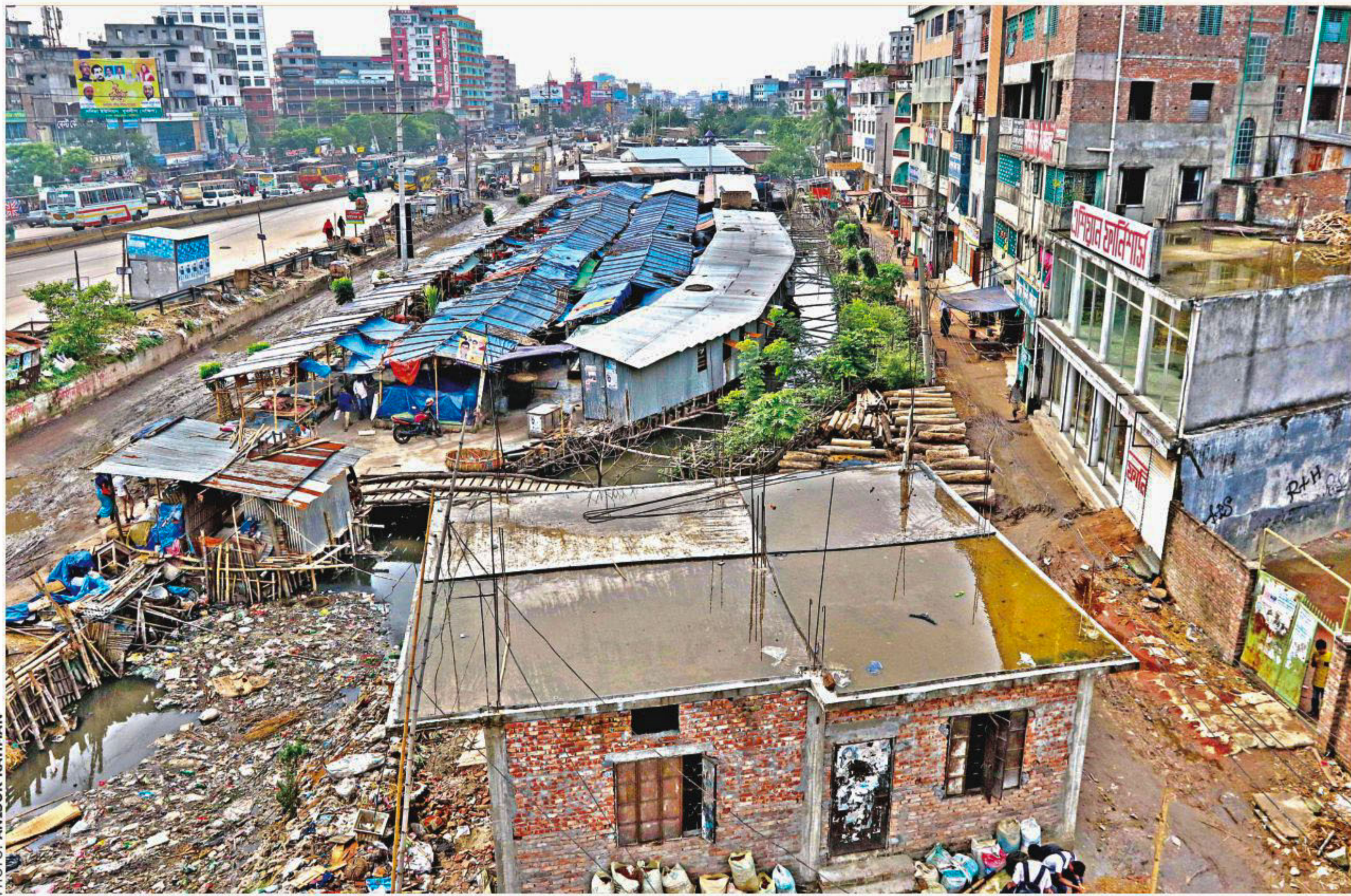
Encroachment chokes off the DND canal in the capital's Jatrabari area. Businesses have occupied a major part of it to set up shops, kitchen markets and other illegal erections obstructing the flow in the canal. Perennial water-logging during the rainy season makes life in the area miserable. The photo was taken yesterday.
