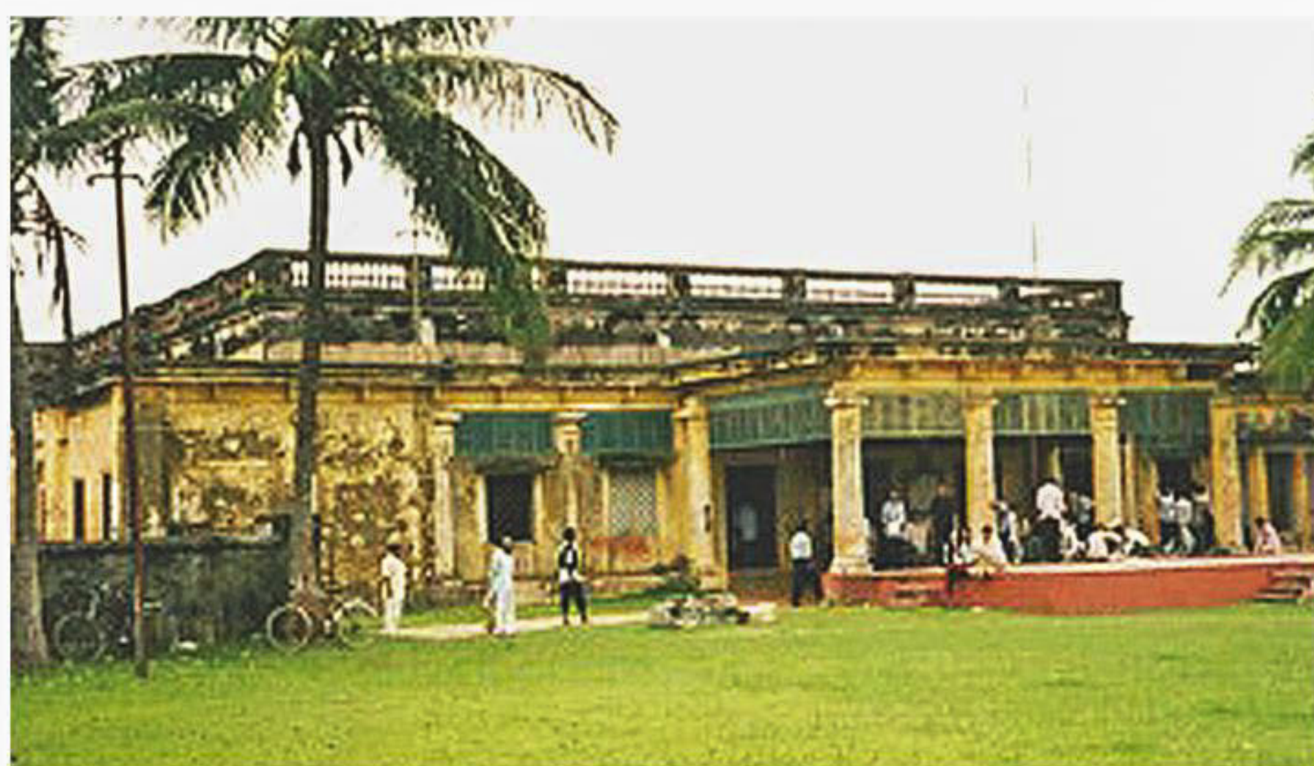
The 17-room Palmer House - now the Purnea College in Bihar, today. The building is still in a fairly pristine condition
