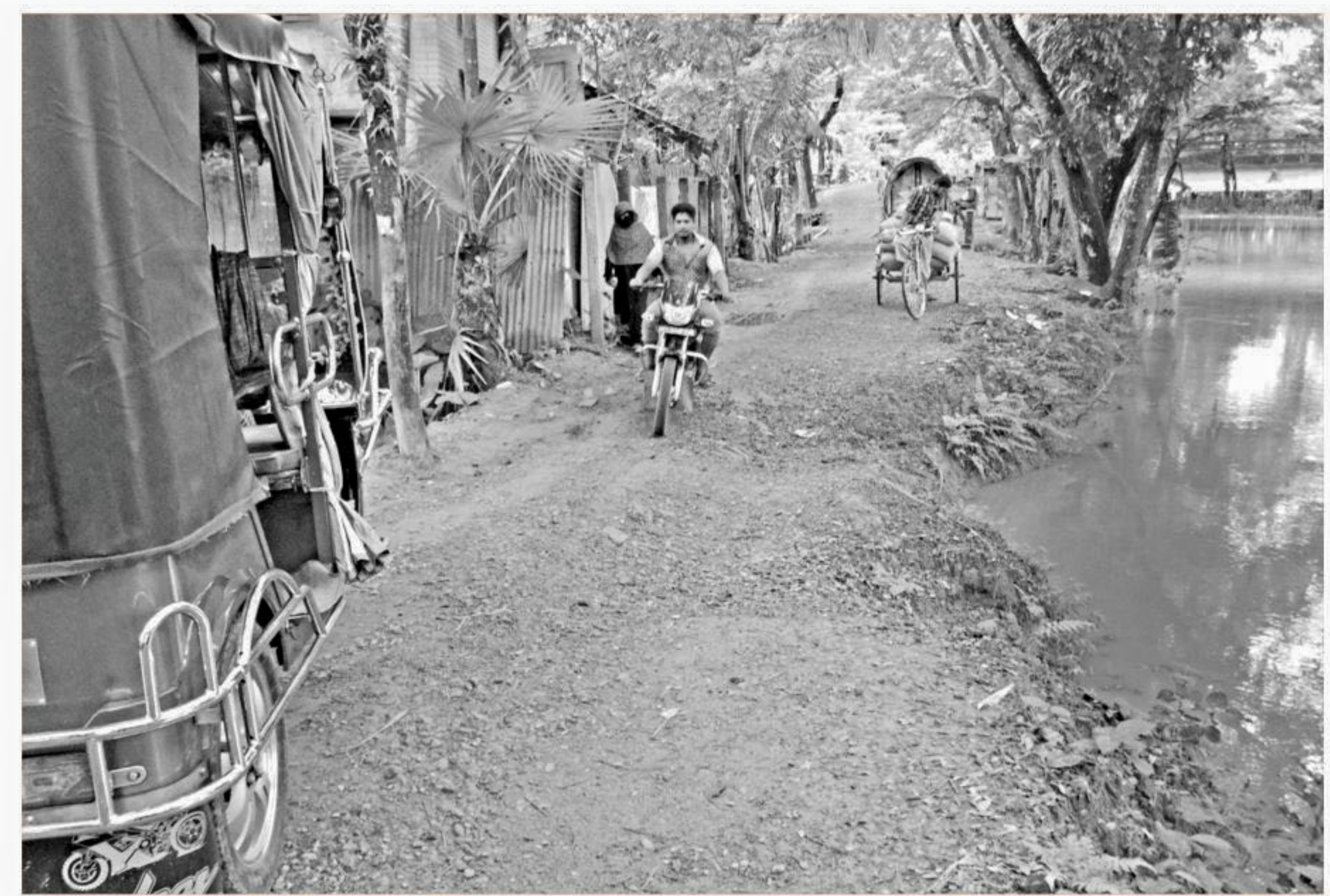
The five-kilometre road from Pukurijana to Mankisundar in Rajapur upazila under Jhalakathi district remains in an awful state for years, much to the nuisance for commuters. The photo was taken from Pukurijana a couple of days ago.
