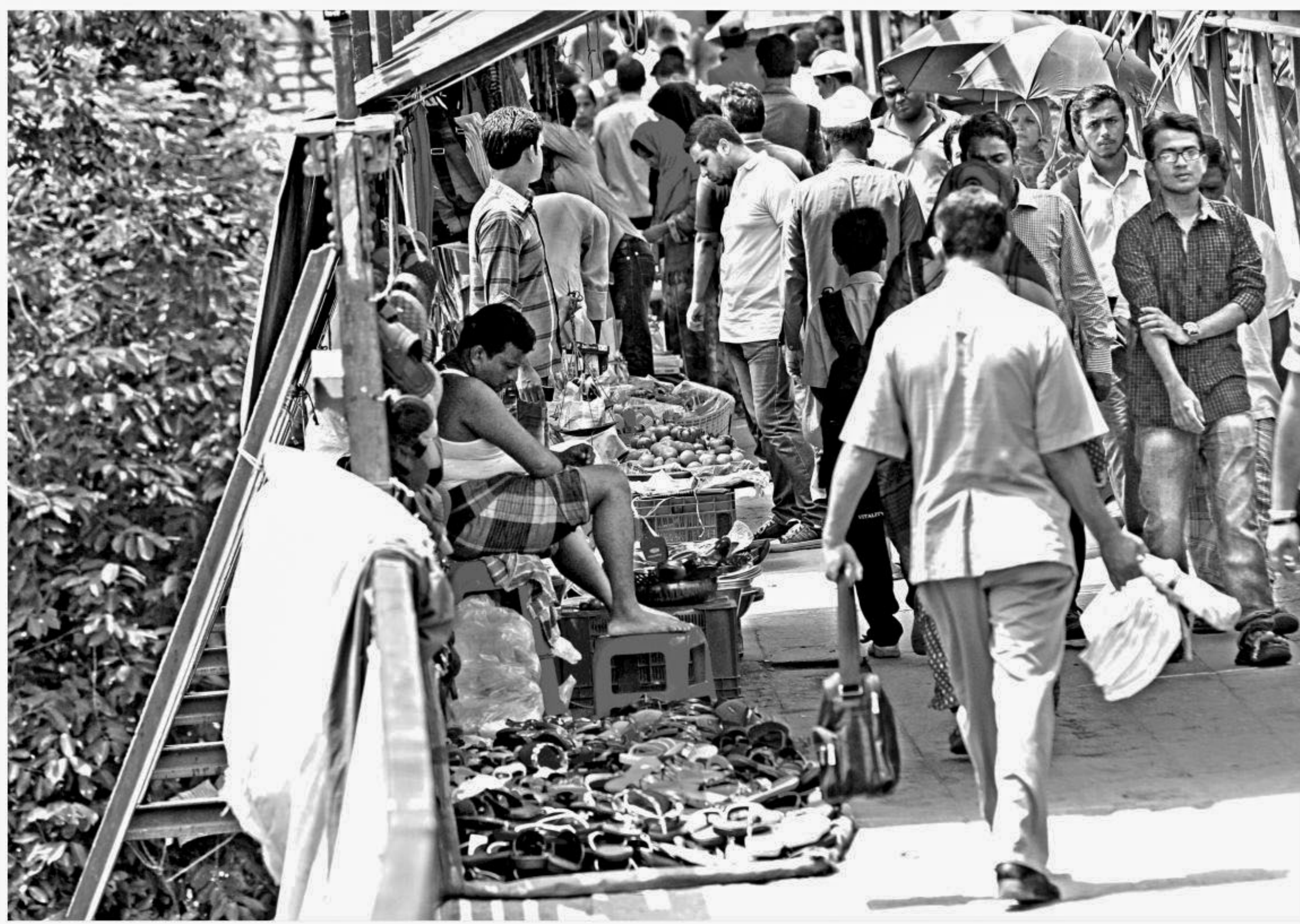
Hawkers and vendors keep exploiting a considerable portion of the footbridge over the capital's Kamalapur Railway Station for their own benefits, forcing commuters to suffer. The photo was taken yesterday.
