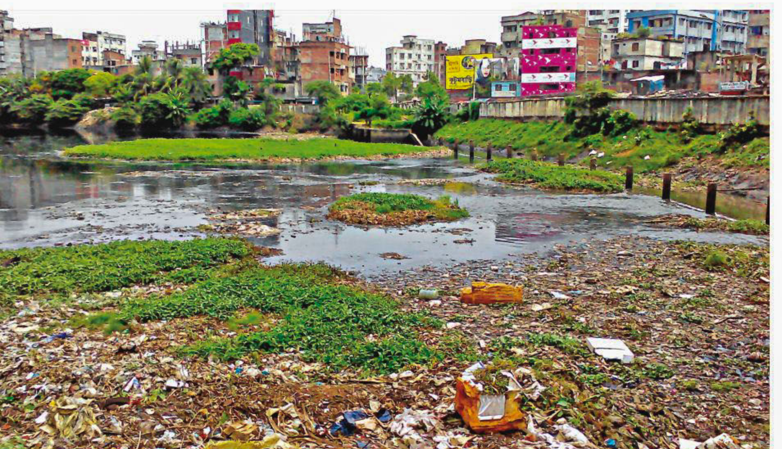
Dholai Khal retention area narrowed down for construction of a box-culvert.
