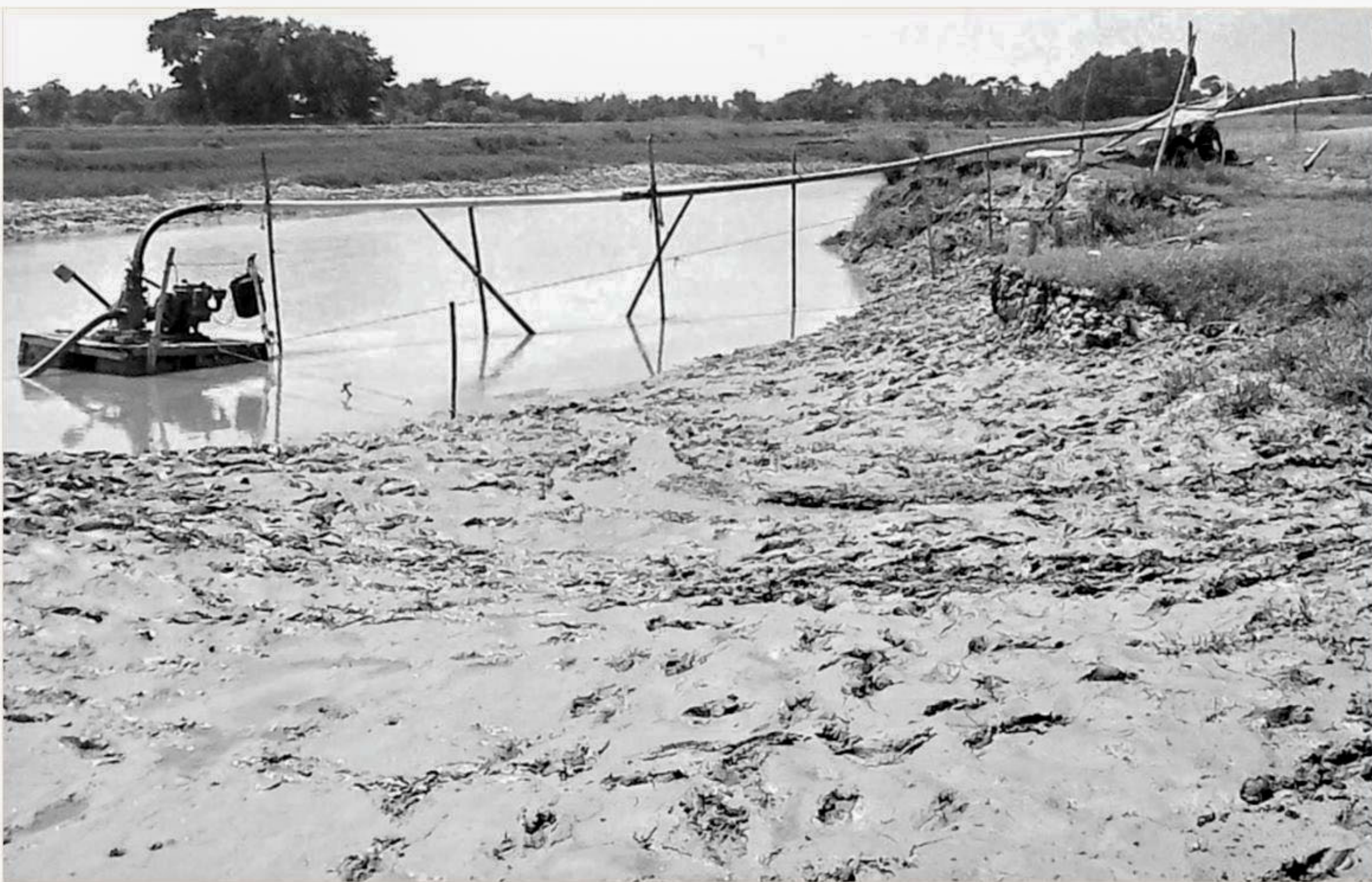
Illegal lifting of sand by shallow machines from Laghata River in Potonushar union under Kamalaganj upazila of Moulvibazar is going on unchecked, posing a threat to agriculture and the people of the area.
