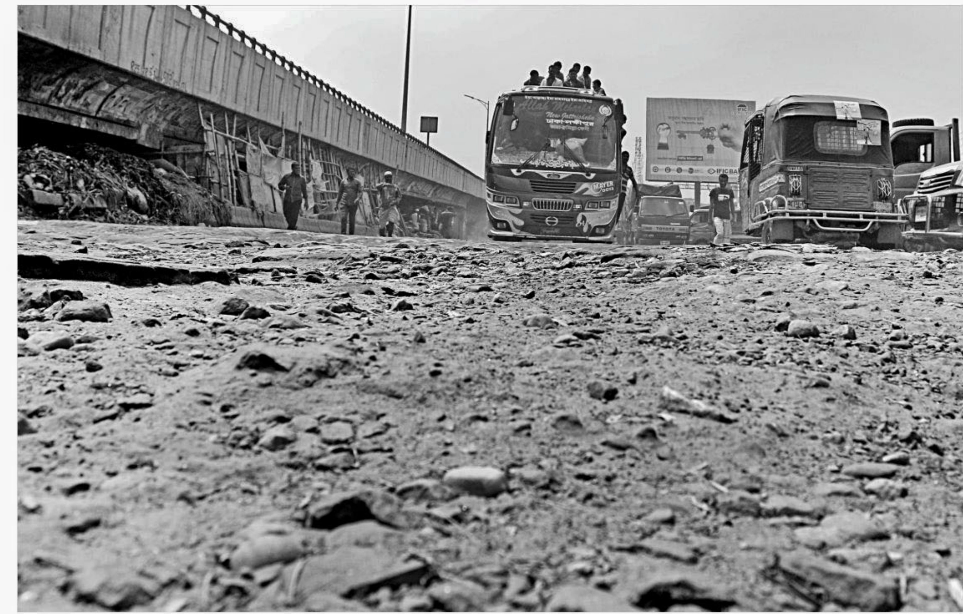
The road under Mayor Mohammad Hanif Flyover near the capital's Demra area is in a terrible state, mainly due to a lack of proper maintenance. The asphalt is gone and the road is plagued with potholes, making it difficult for vehicles to pass through. The photo was taken yesterday.
