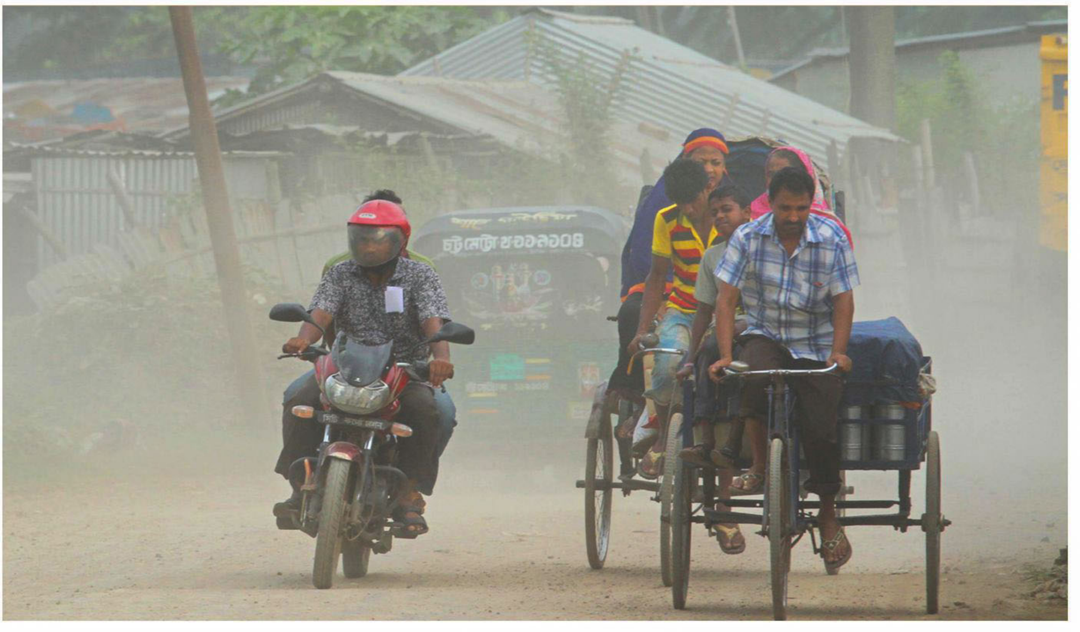
Commuters face suffocating dust while travelling the worn out Signal Ghar road in Haliashar area of the port city. Road dust due to unplanned digging of roads for installing utility lines and lack of proper repairment has become a major source of air pollution causing health hazards to the city dwellers. The photo was taken on Tuesday near Chittagong Women Polytechnic Institute.
