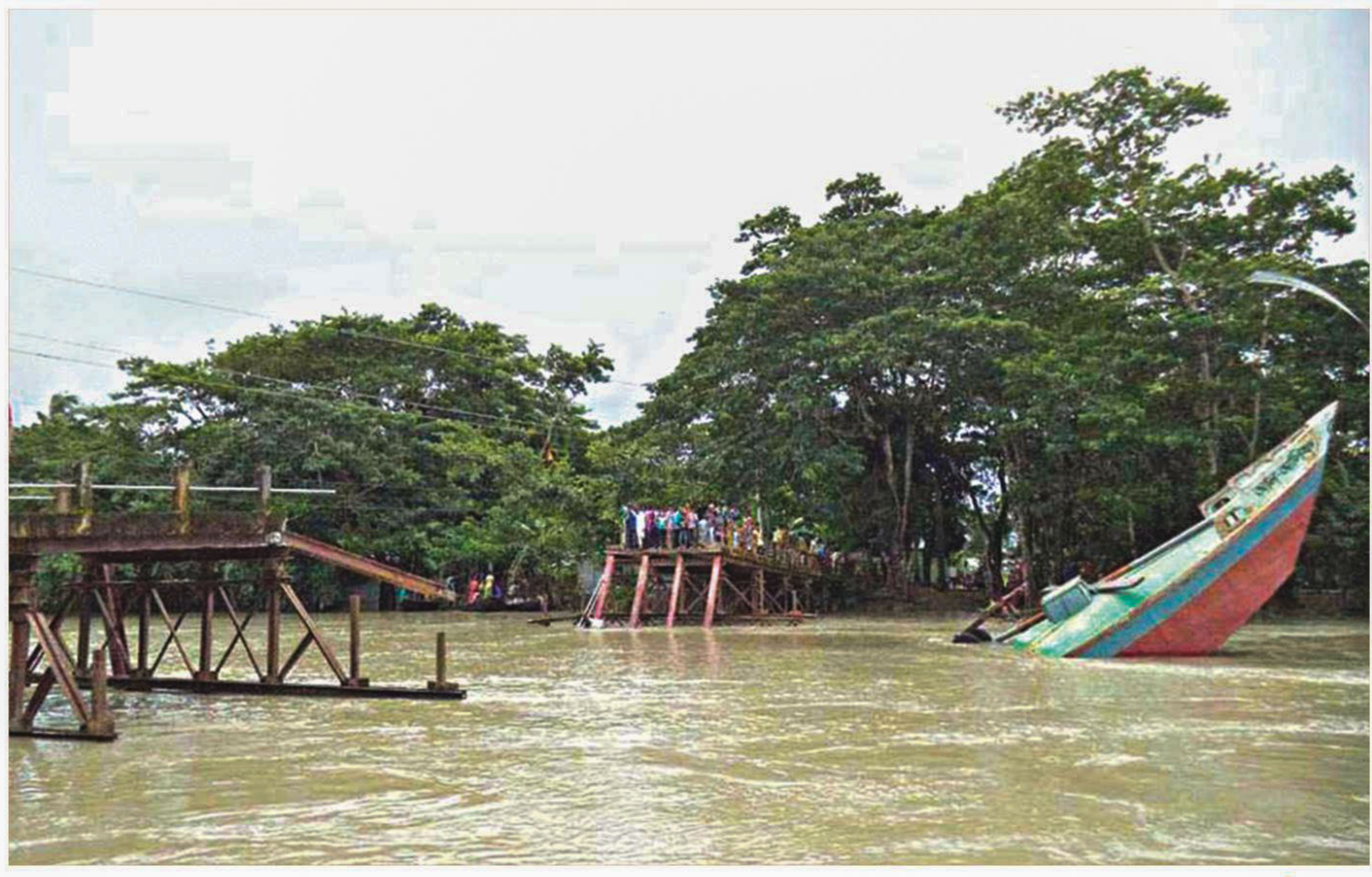
A large section of an iron bridge at Amua in Jhalakathi's Kathalia upazila collapsed yesterday after being hit by a sand-laden cargo vessel. The bridge is essential for the locals to go to Amua Hospital -- the only one available in the upazila.
