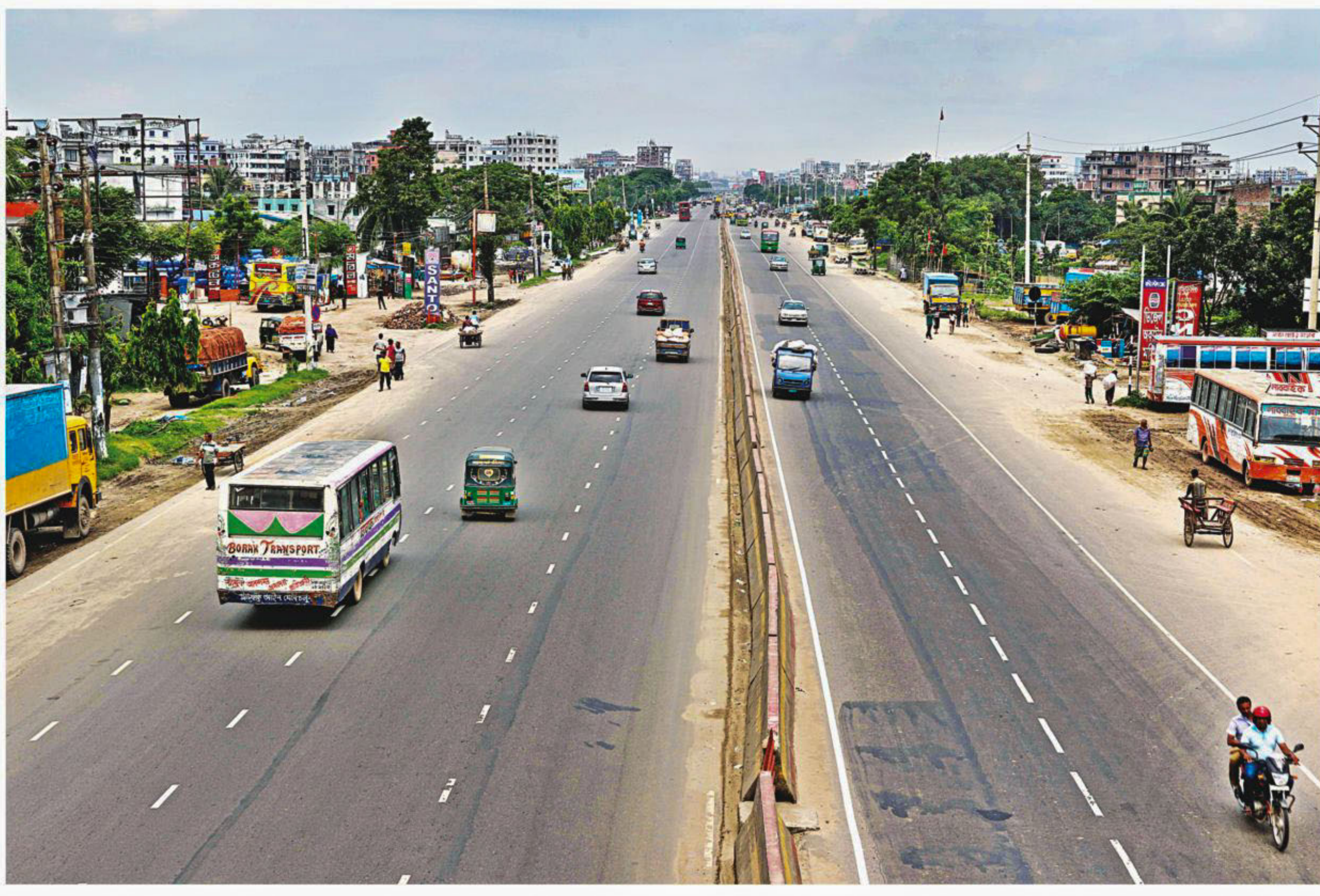
The country's first eight-lane highway corridor, from Jatrabari to Shimrail, which Prime Minister Sheikh Hasina will inaugurate today. The prime minister will also open the construction of the country's first four-lane expressway today. The photo was taken at Shonir Akhra in the capital yesterday. PHOTO: STAR
