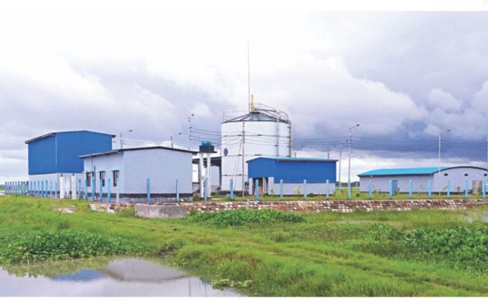
A view of straw-based bio-gas cum power plant, the first of its kind in the country, at Bashbaria in Dashmina upazila under Patuakhali district. PHOTO: STAR
