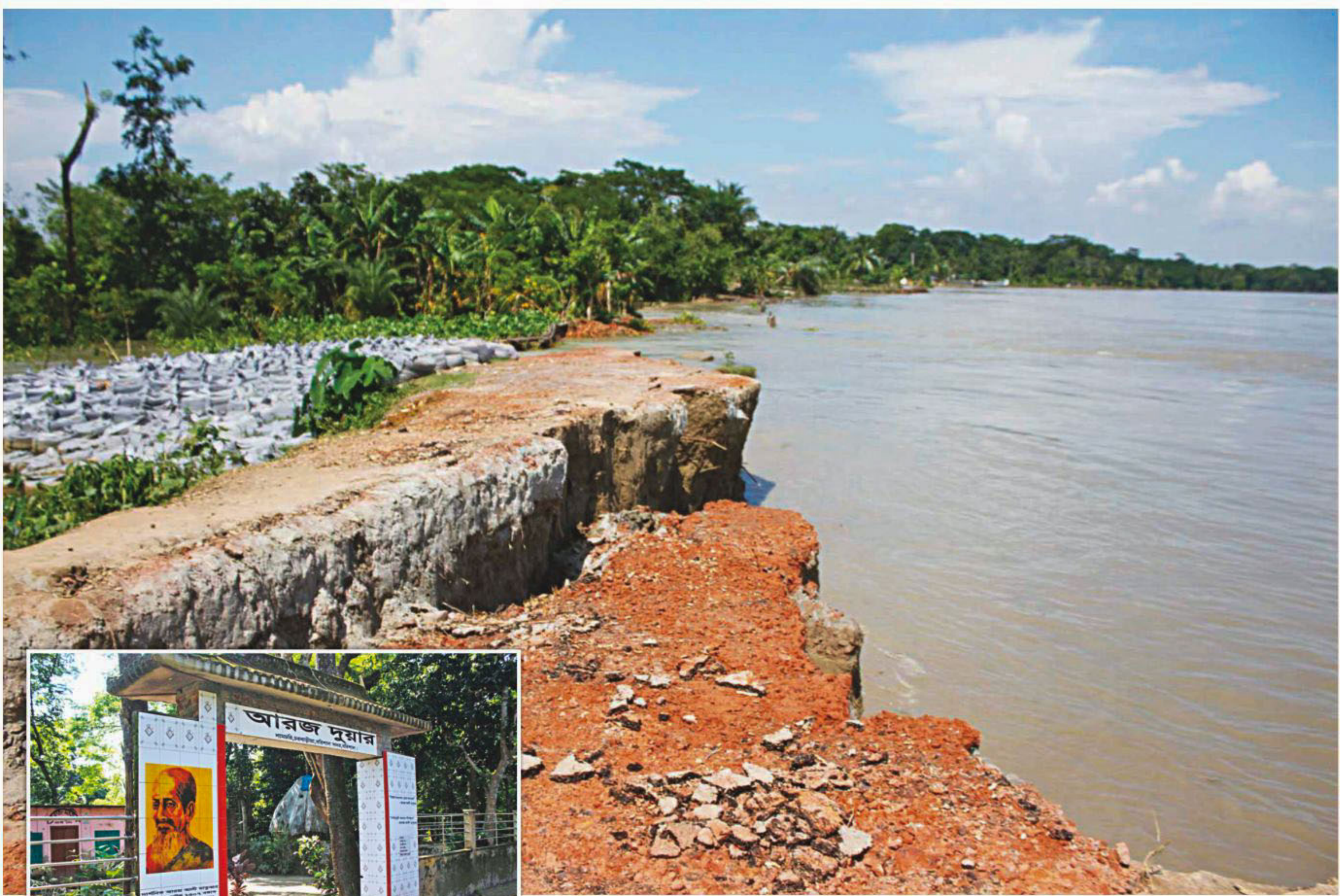
Erosion by the Kirtonkhola River has taken a serious turn, devouring around a kilometre area of the Charbaria-Lamchari road in Barisal Sadar upazila during the last one month. Inset, Aroj Manjil Public Library will also be under threat if urgent protection measures are not taken to check the menace.
