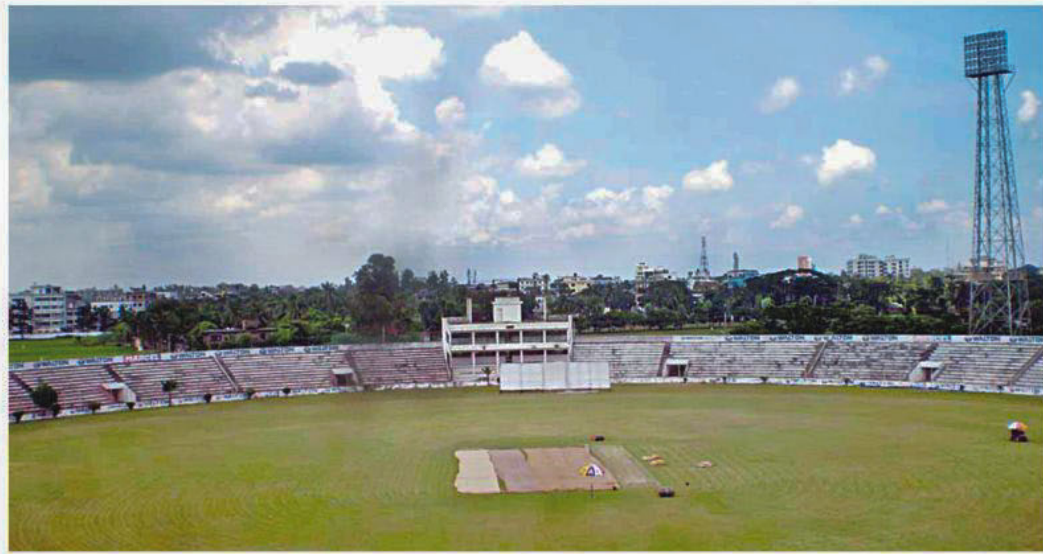
Once a venue that hosted five passionately attended ODIs and one buzzing Test, for much of the past 10 years the Shaheed Chandu Stadium in Bogra has become host to foliage growing through cracks in the neglected galleries in the absence of any international engagements. PHOTO: STAR
