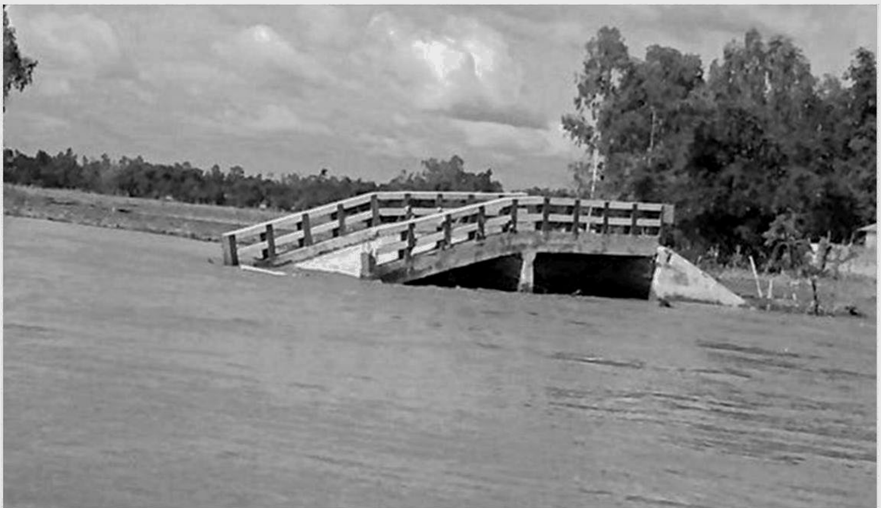
The bridge that collapsed recently due to strong current of the swelling Teesta on Teesta Bazar-Ekotar Bazar road in Dimla upazila under Nilphamari is still under water.
