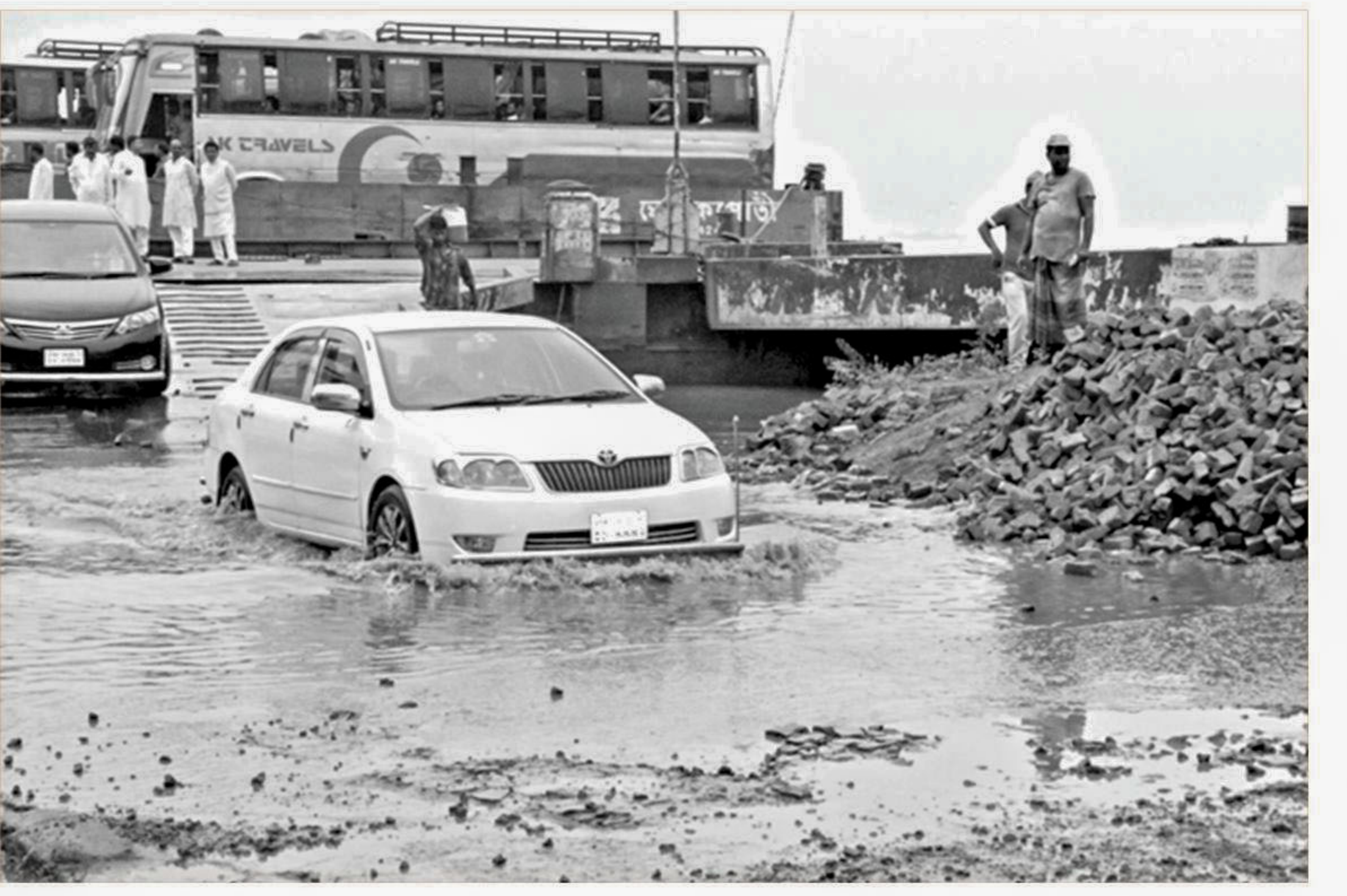
Vehicles move through water as erosion by the Padma River damages two landing stations of Daulatdia ferry terminal in Manikganj. PHOTO: STAR
