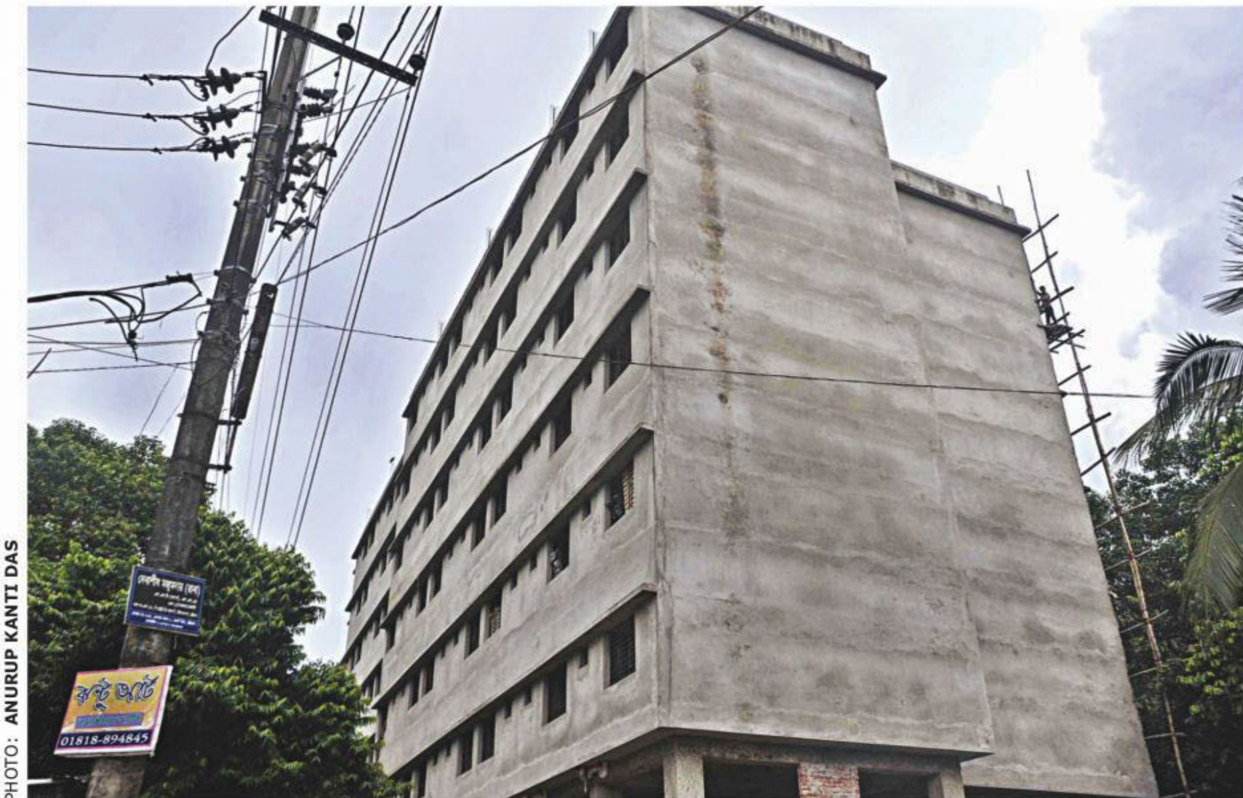
PHOTO: ANURUP KANTI DAS The building constructed by Chittagong City Corporation in Tigerpass Batali Hill area was supposed to be a home for poor families living at risk of landslides in the hillside slums, but the authorities are now overturning their decision, reasoning that the pledge made by the administration of ex-mayor M Manjur Alam was not pragmatic.
