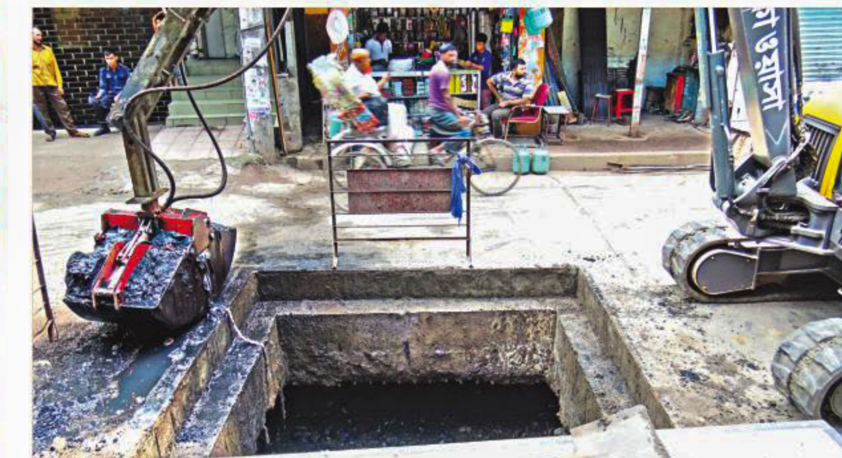
City corporation cleaning a box culvert in Segunbagicha.
