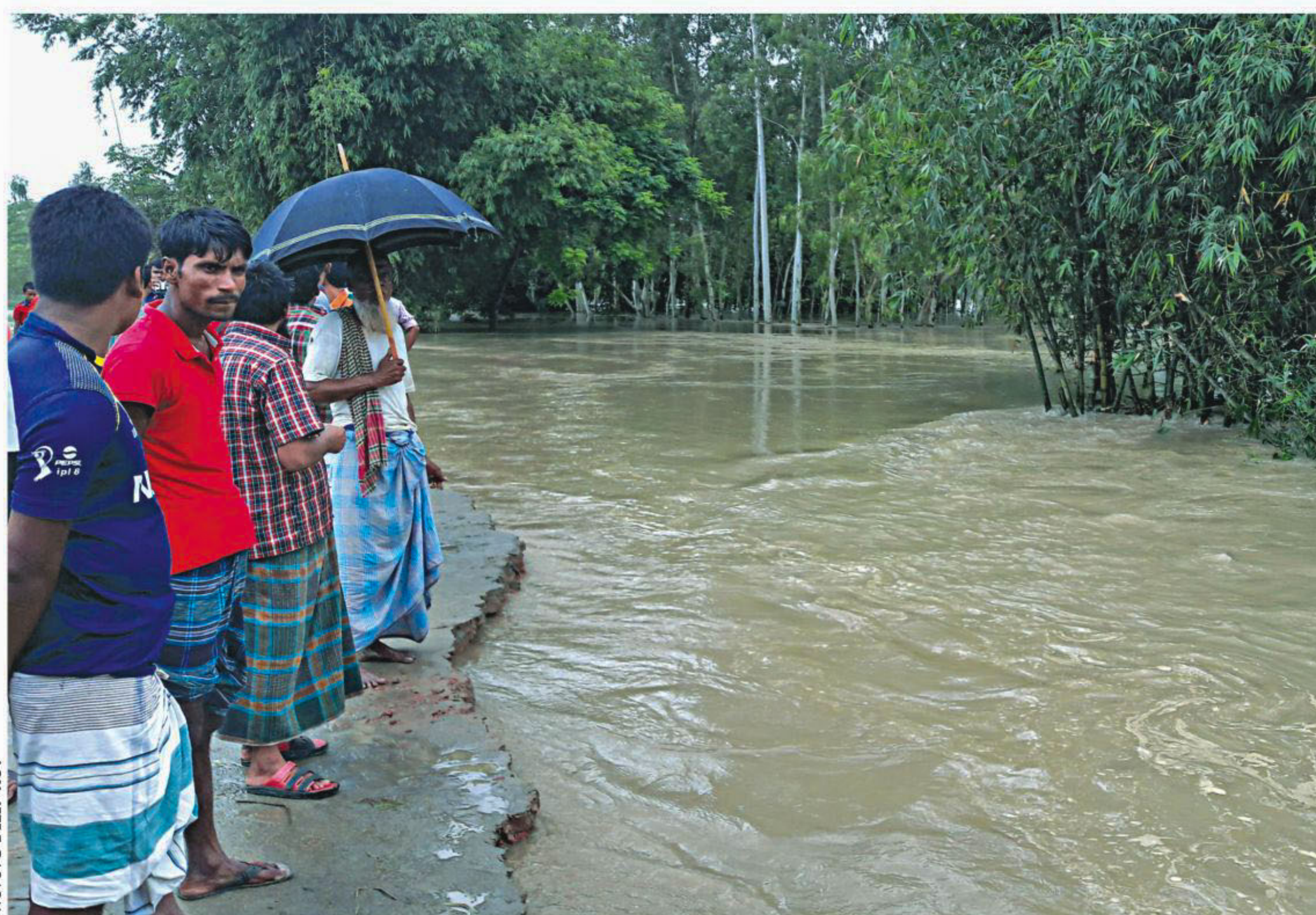
People stand on the edge of badly damaged 120-metre dam of Water Development Board at Shiberkuti village in Lalmonirhat Sadar upazila. Heavy water flow from the Dharla river washed away a big chunk of the dam, inundating six villages in the upazila. The photo was taken yesterday.
