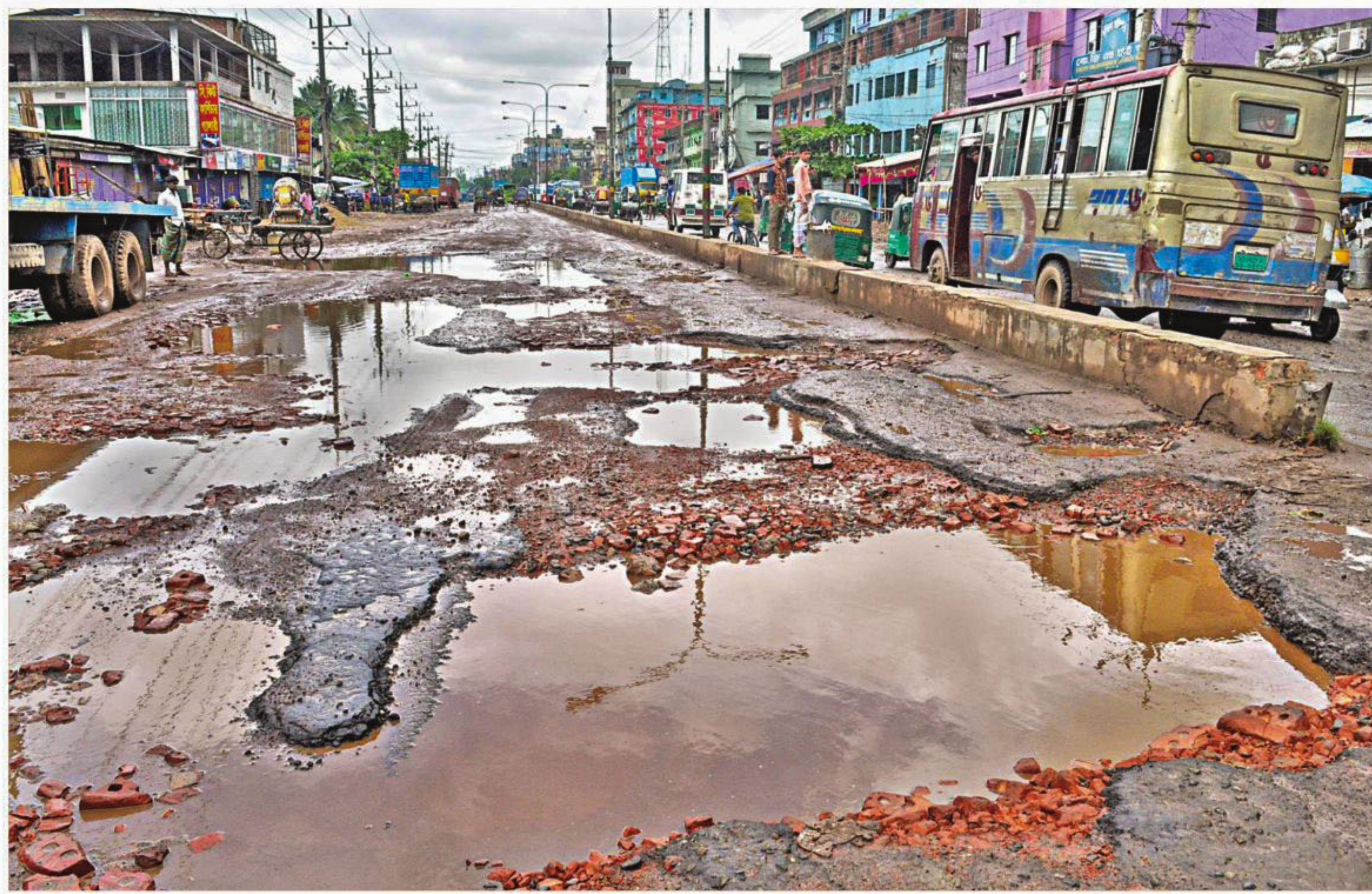
With potholes and craters developing in many of the port city roads as the rains continue to drench it for a couple days, travelling in those areas has turned into a nightmare. The photo was taken on Monday in Steel Mill area.
