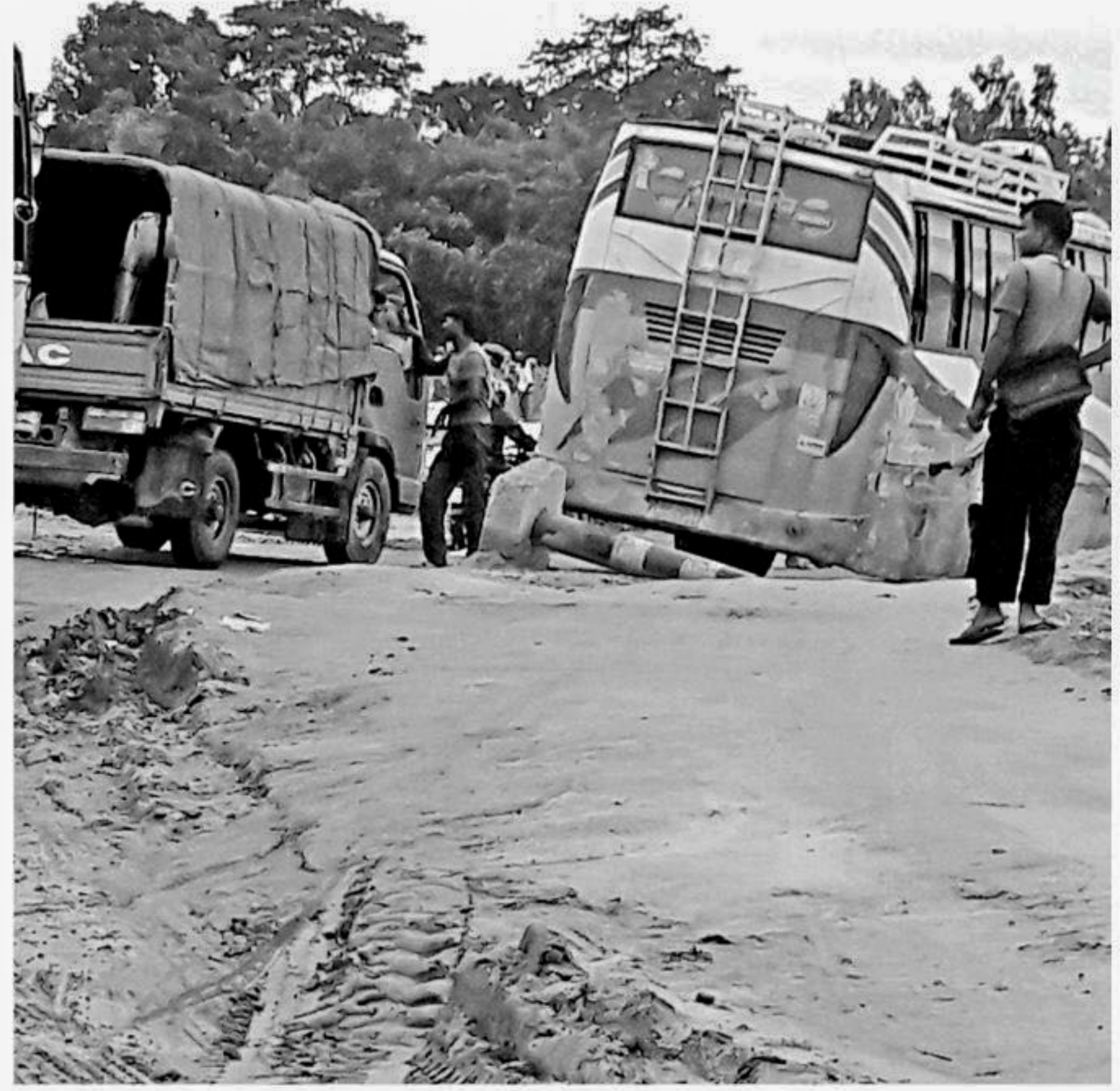
Plying of heavy vehicles over this weak Bailey bridge across the Swarnamati River on Lalmonirhat-Burimari highway poses the risk of serious accident anytime.
