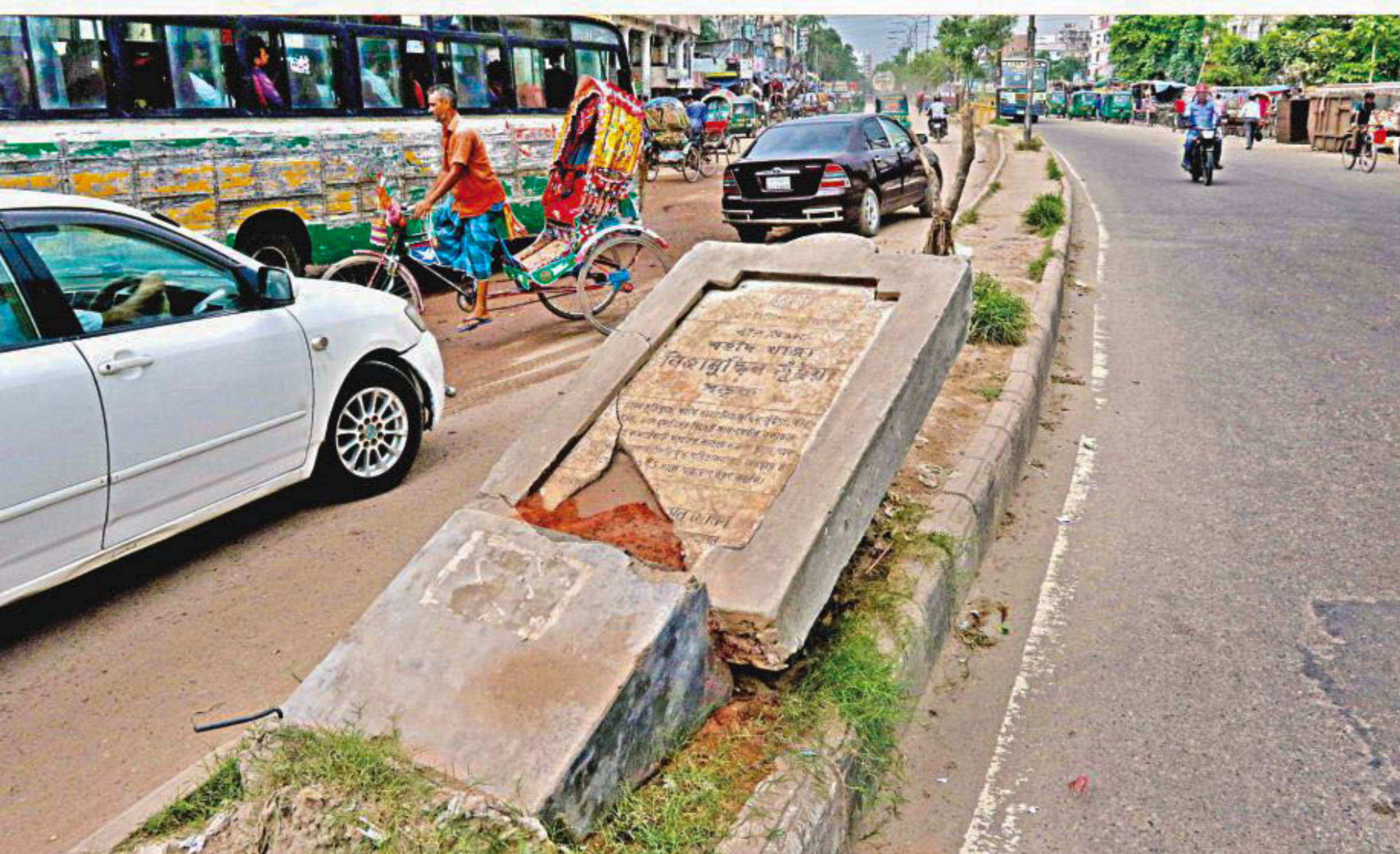
Inaugurated a couple of months ago by the mayor of Dhaka South City Corporation, this plaque now lies in ruin, making it nearly impossible for passers-by to know that this road heading towards Shahjahanpur from the Malibagh rail crossing in the capital was named after Bir Uttam Shaheed Khwaja Nizamuddin Bhuyan, who embraced martyrdom at Atgram Road in Kanaighat thana of Sylhet on September 4 during the 1971 Liberation War. The photo was taken yesterday.
