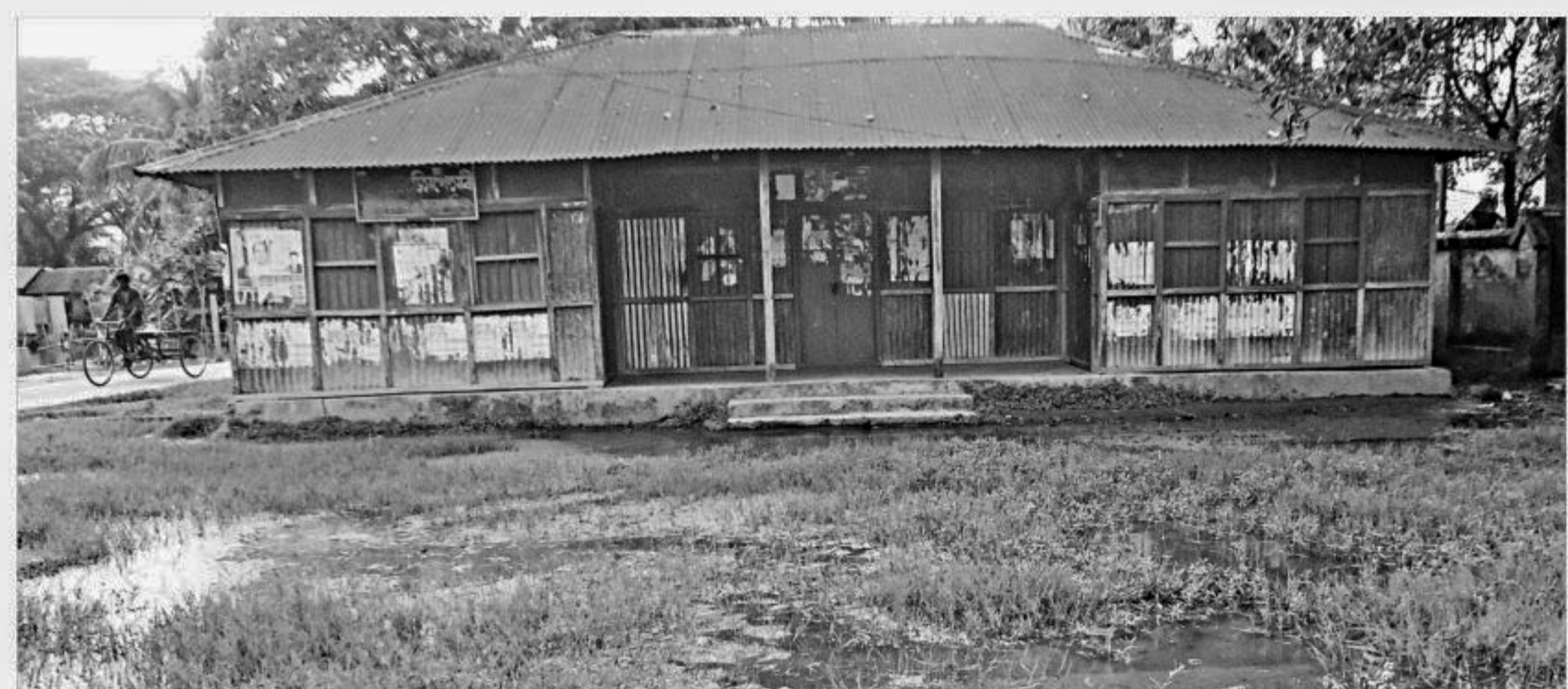
The century-old Phulbaria Dispensary.
