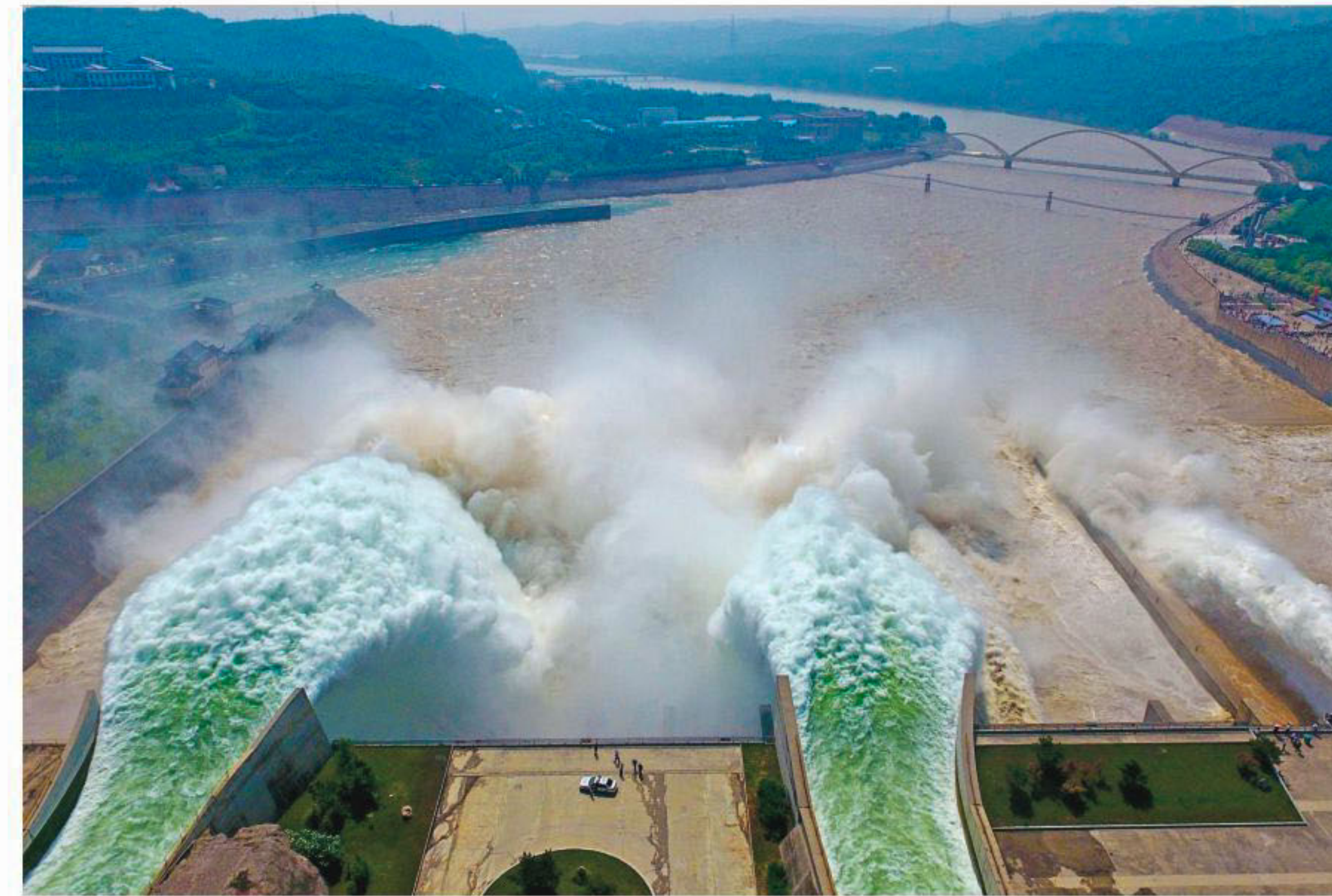
Water is released from the floodgates of the Xiaolangdi dam on the Yellow River near Luoyang, in China's Henan province, yesterday. The floodgates are opened every year in an operation to flush millions of tonnes of silt from the river bed.
