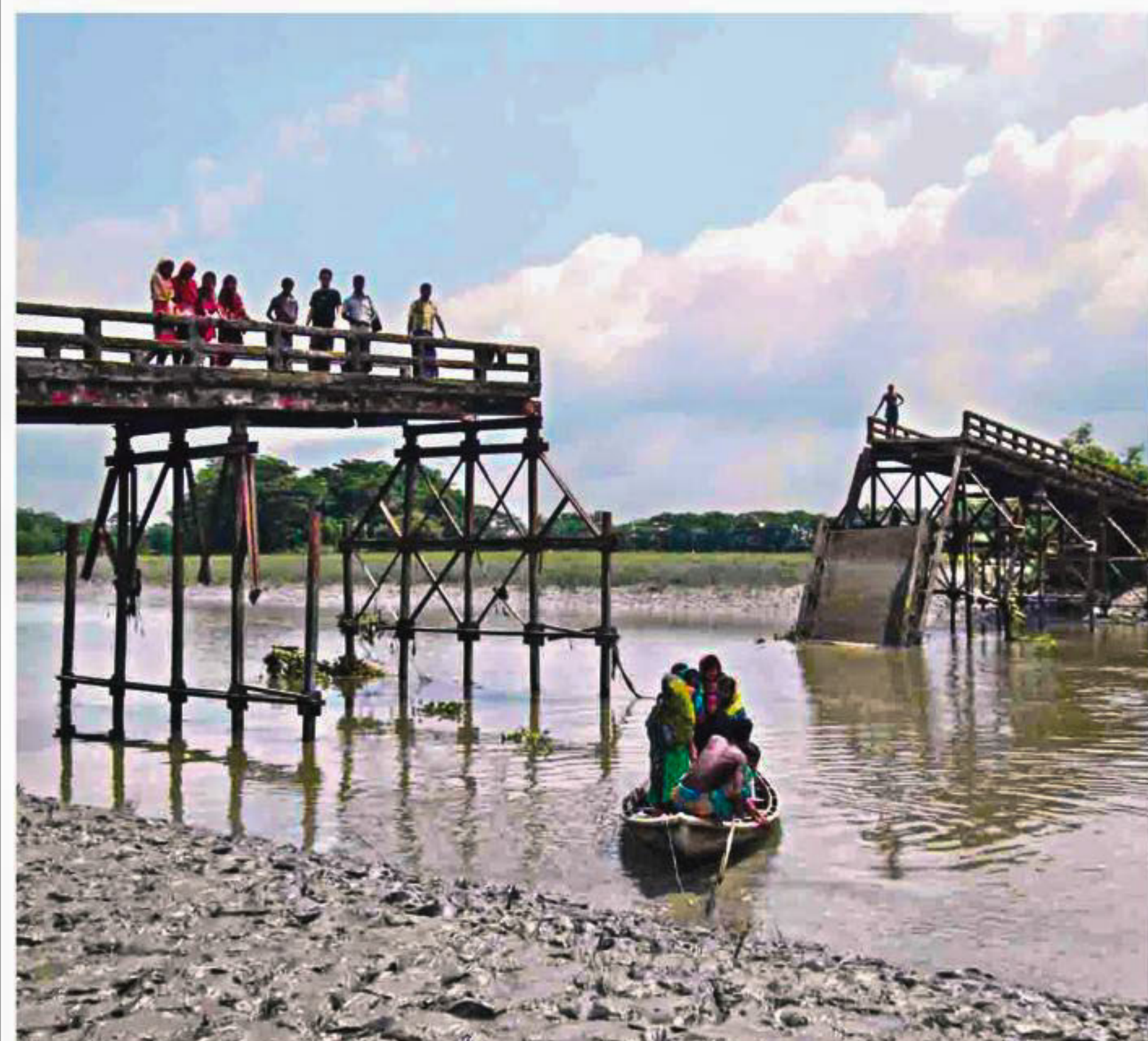
Collapsed during cyclone Roanu on May 21, this bridge over Banshbnunia canal in Amtali upazila under Barguna district is in need of urgent repair or reconstruction to mitigate sufferings of thousands of people in the area.
