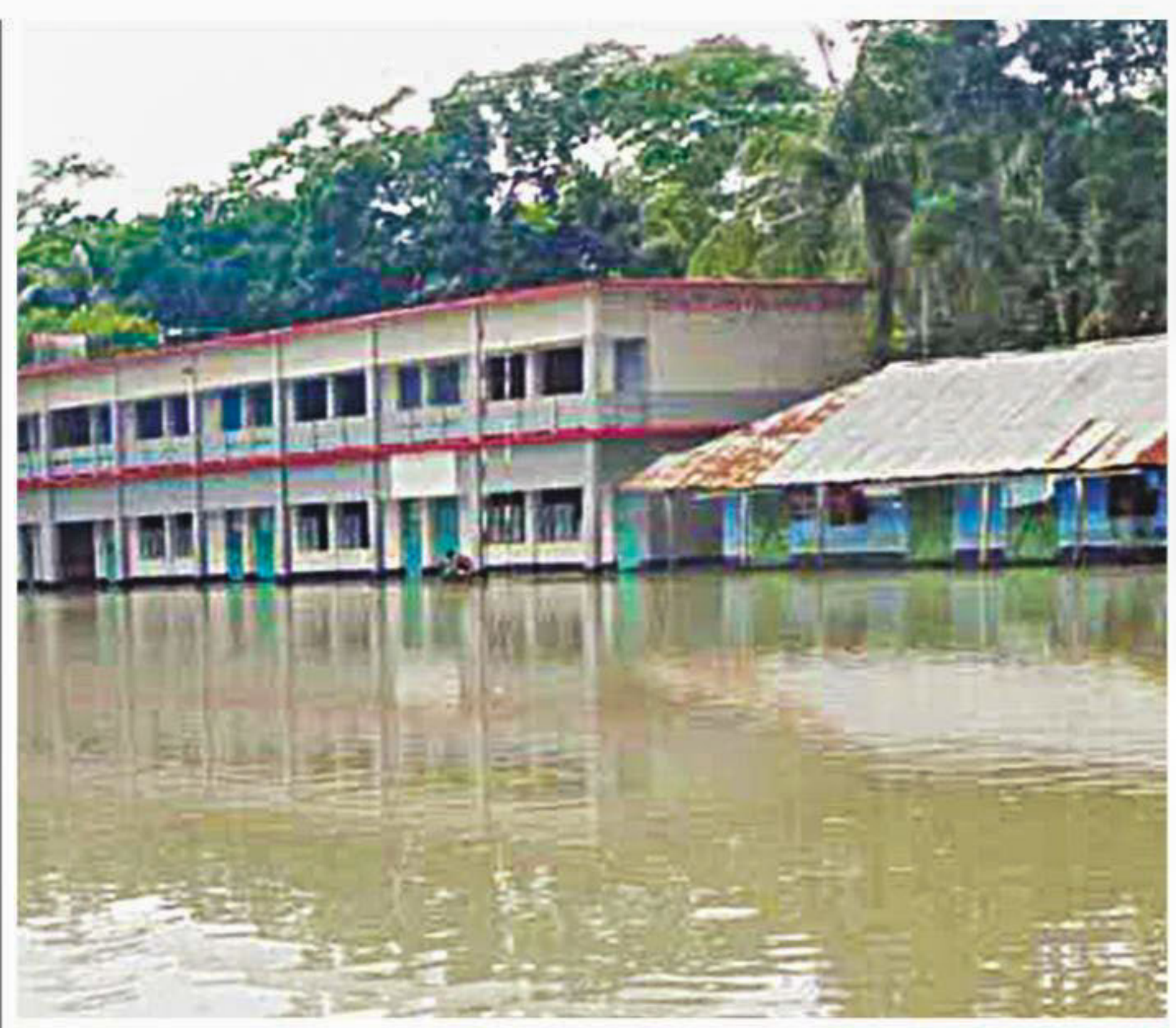
Five villages in Patuakhali's Mirzaganj upazila get flooded following collapse of Payra River's dyke at two points under the pressure of tidal water yesterday. Photo shows the submerged playground of Mirzaganj Darbar Sharif Government Primary School.
