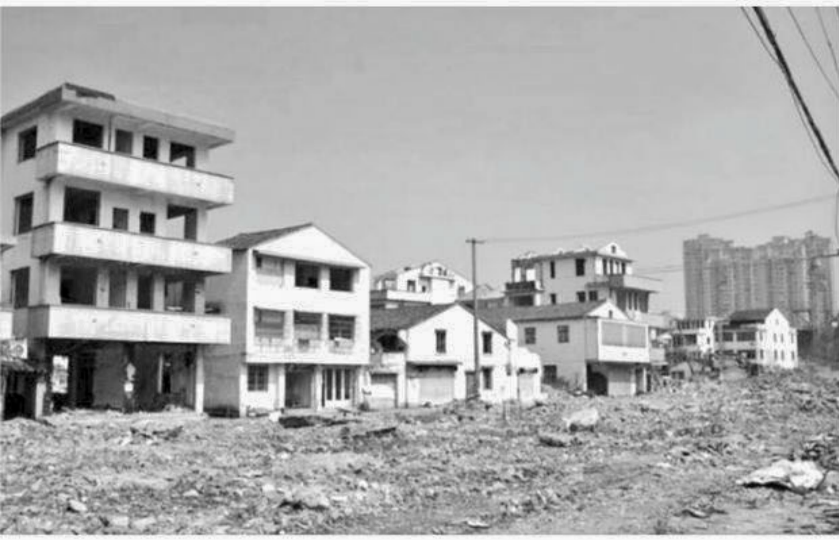
Half-demolished buildings and debris are seen in Wenzhou, China.
