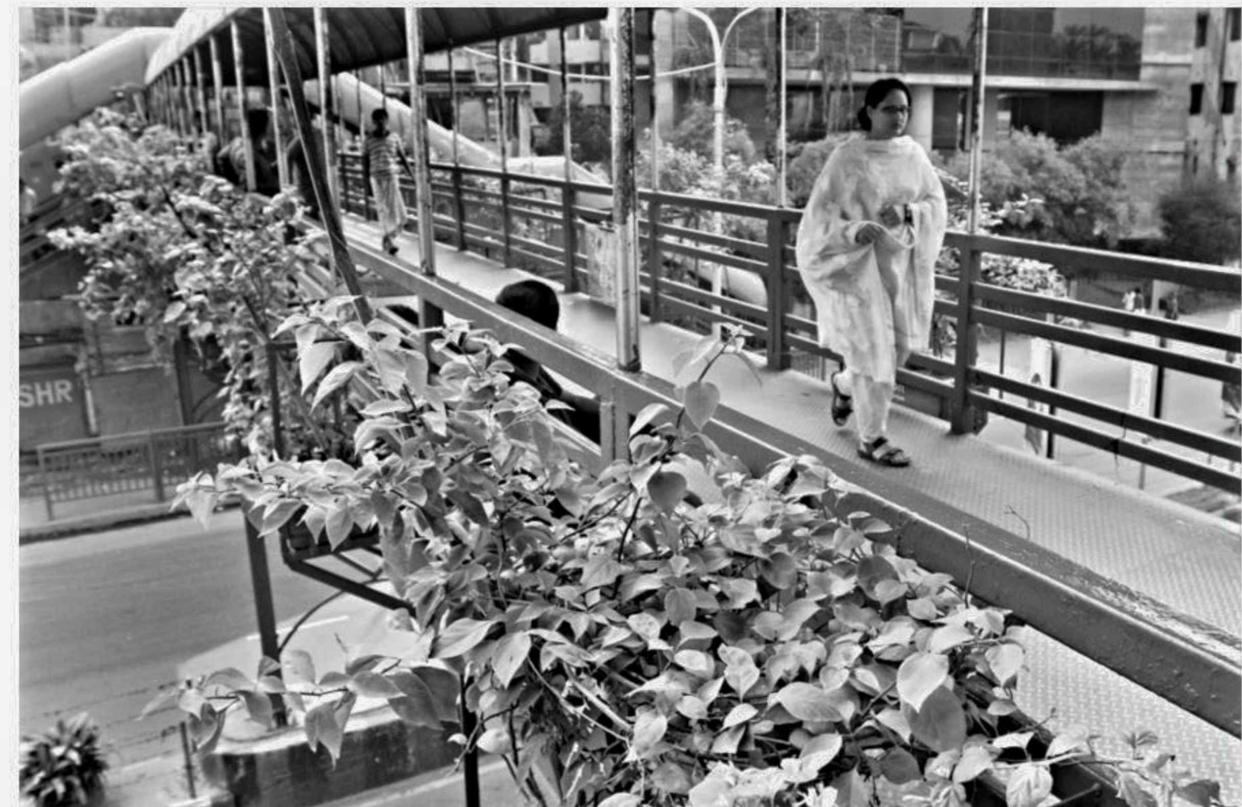
Repainted footbridges - one of the first steps to improvement.
