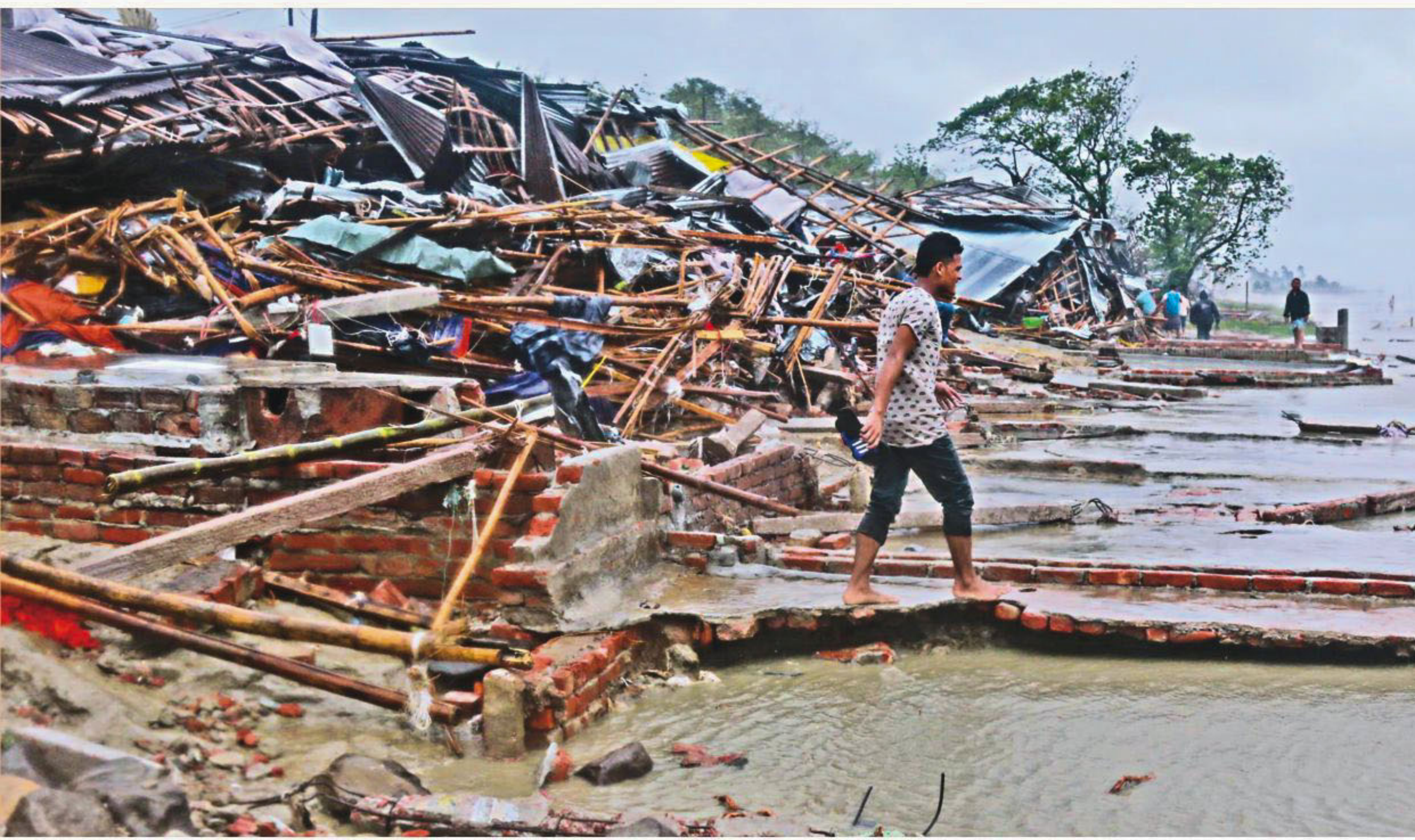
The torn and twisted corrugated iron sheets and bamboo from makeshift stalls on the Patenga Beach in Chittagong after Cyclone Roanu devastated the tourist spot yesterday.
